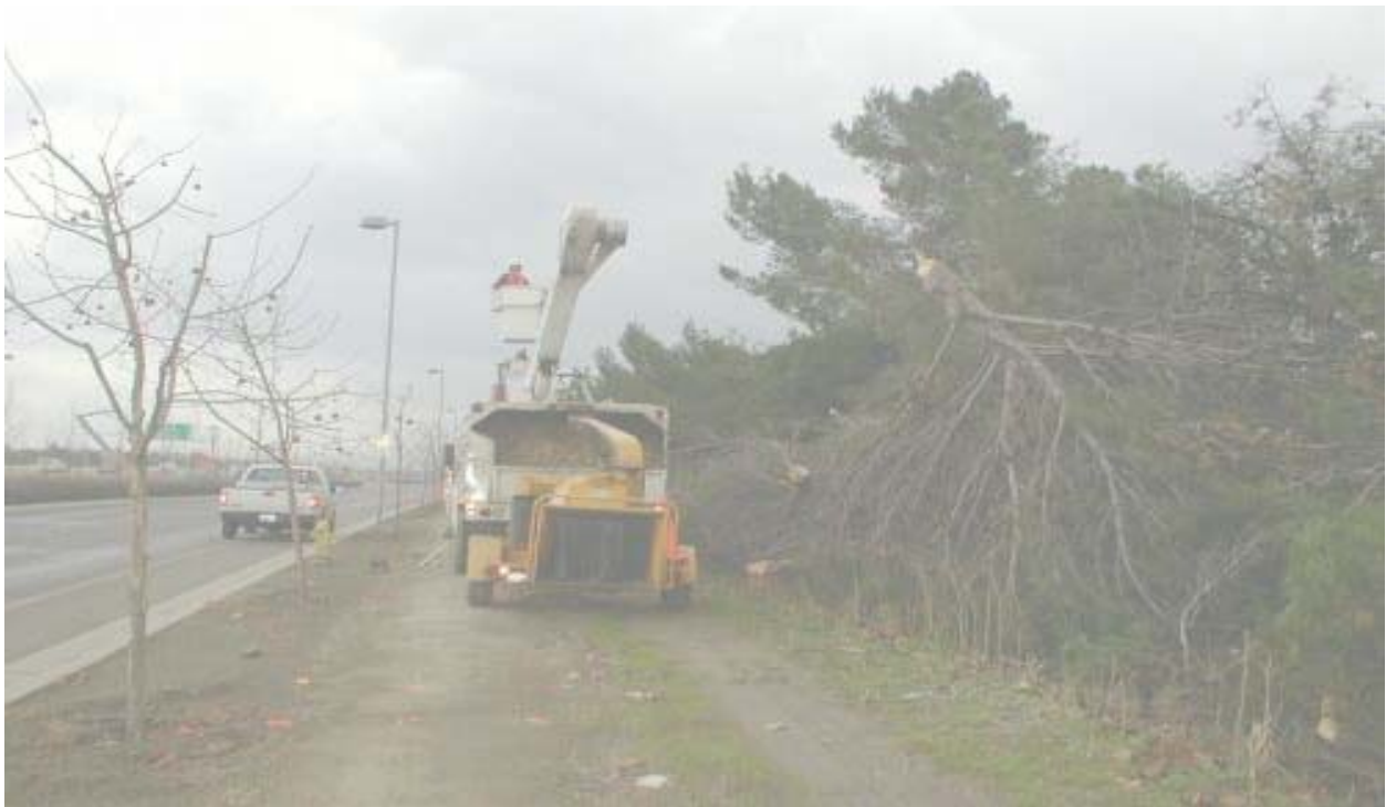
Figure 4 Davey Tree Service Topping Trees Between Pole Foundations #16 and #17 January 9, 2003
