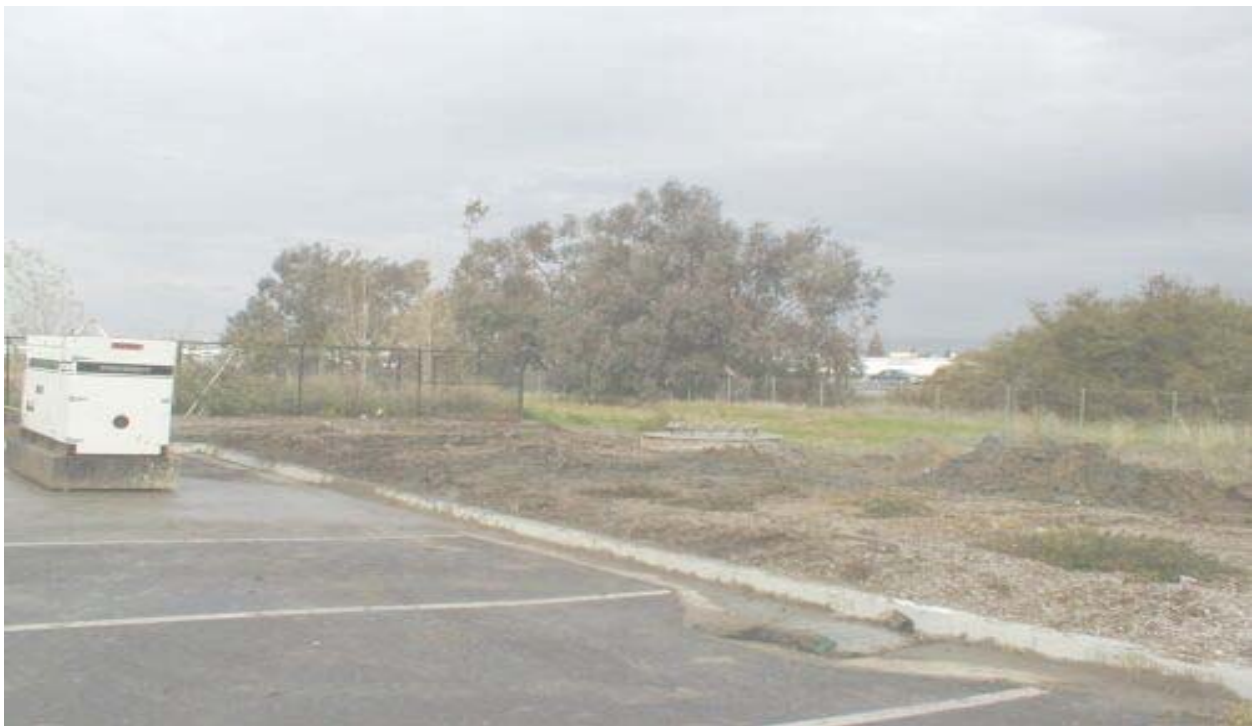
Figure 2 Pole Foundation #3 Completed January 9, 2003
