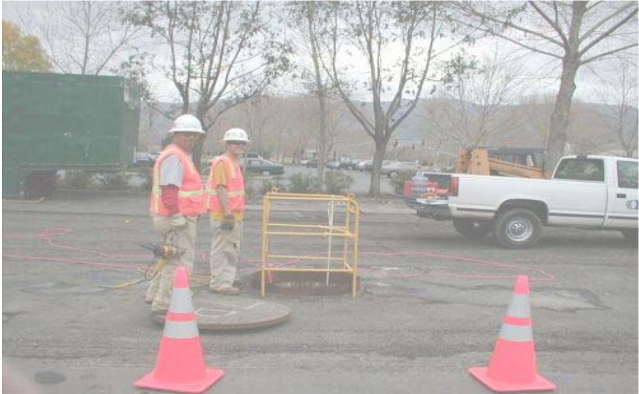
Figure 3 Crews Working on Racking at Man-Hole Vaults #7 January 9, 2003
