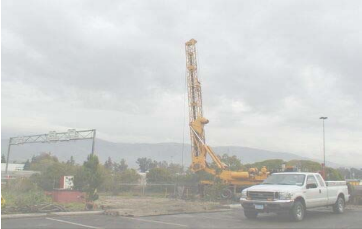
Figure 1 Tri-State Drilling Waiting for Cement Trucks at Pole Foundation #4 January 9, 2003
