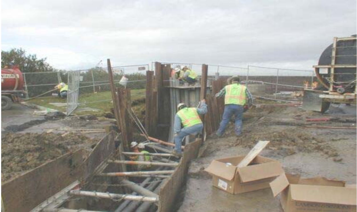
Figure 5 Tie-in for Underground to Overhead at Foundation #9 January 10, 2003
