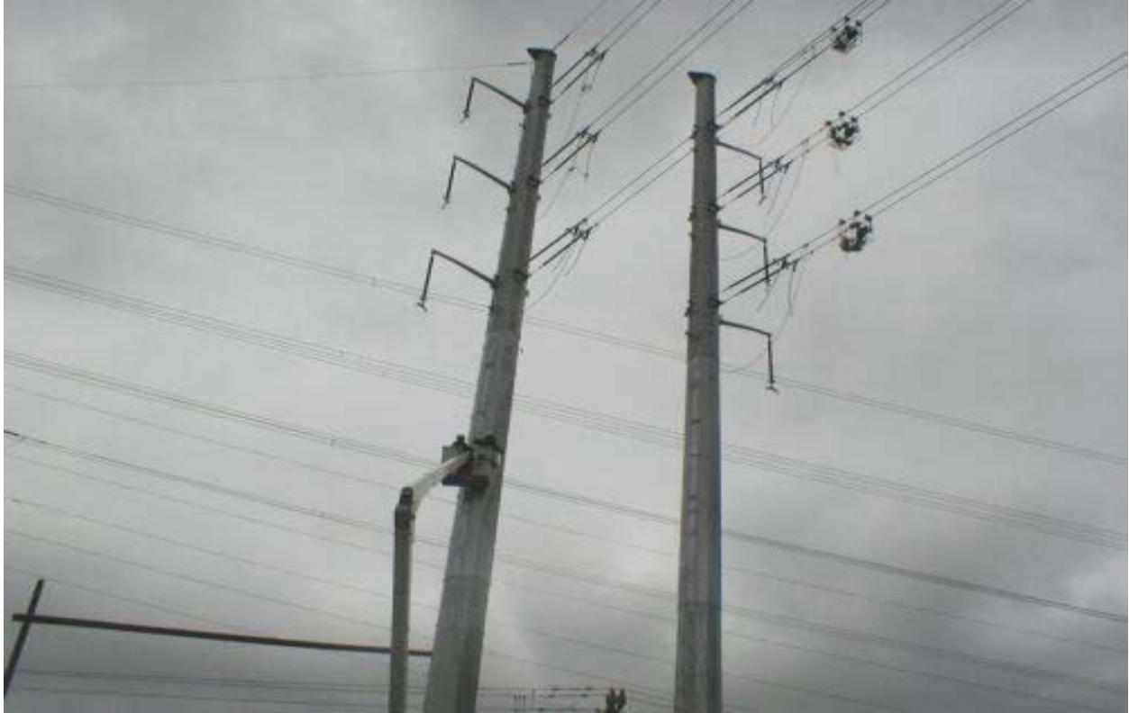
Figure 1 Pole Structure #1(a) and (b) April 2, 2003
