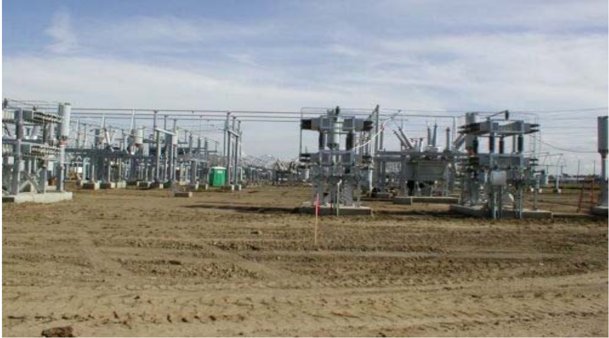
Figure 2 Los Esteros Substation – Recent Grading Work April 30, 2003
