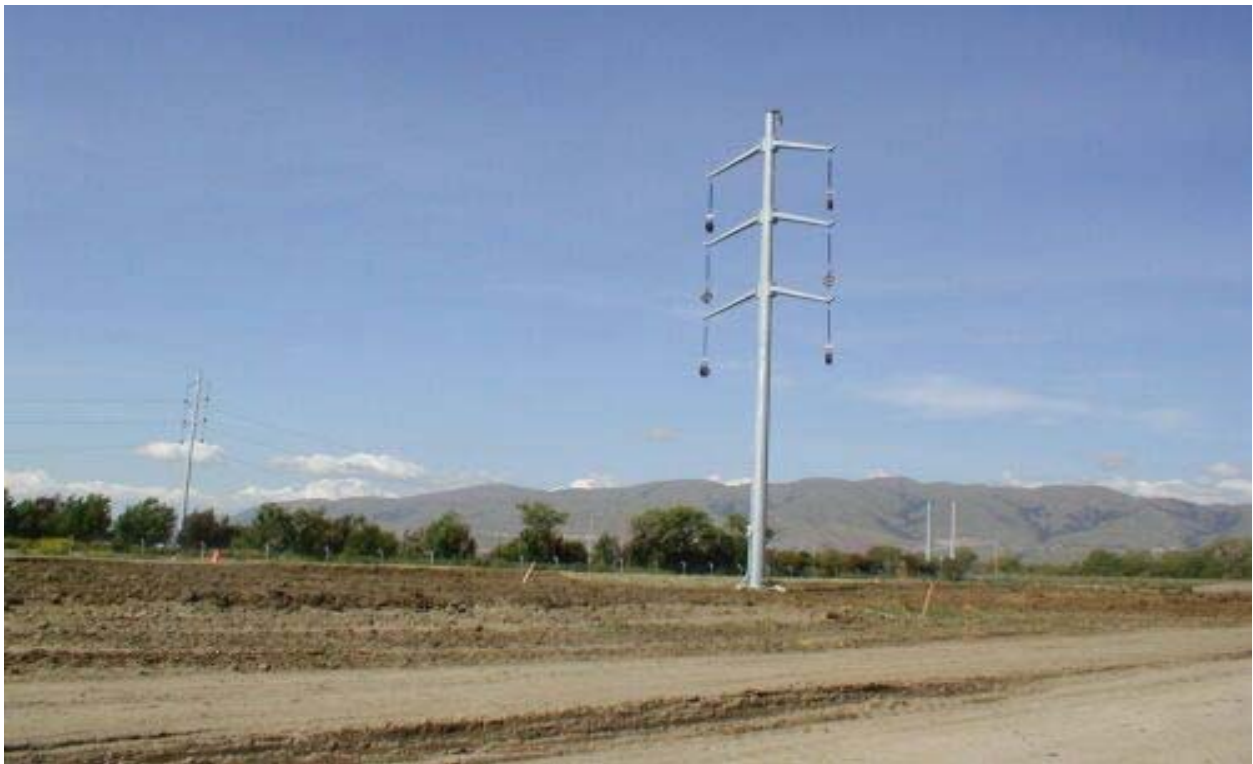
Figure 3 View from Los Esteros Substation Looking Northeast April 30, 2003
