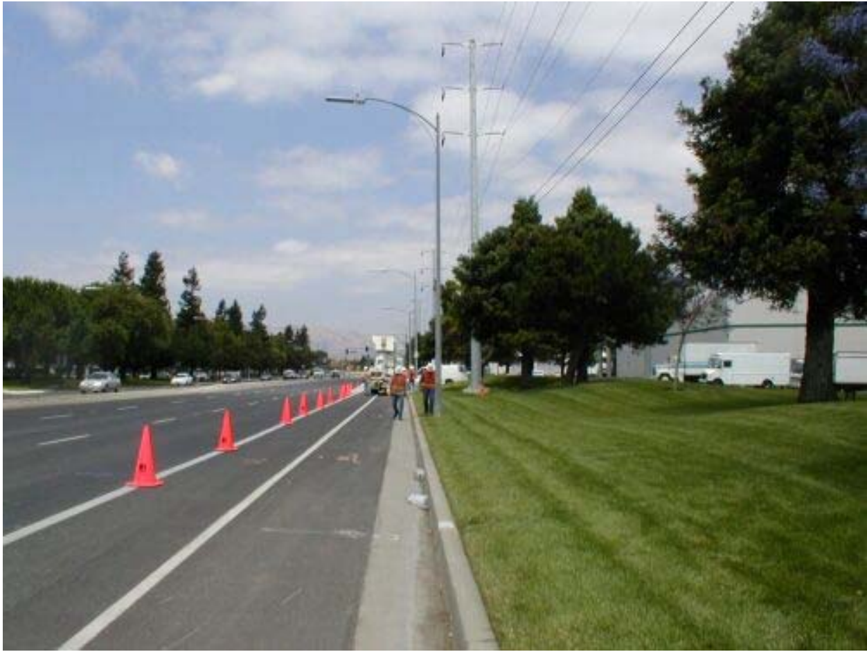
Figure 3 Work Along Trimble Road for the Trimble-Montague Segment June 11, 2003
