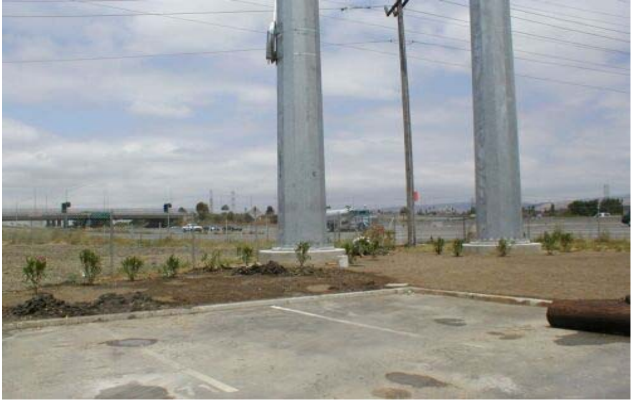
Figure 1 Landscaping Work at Poles #1 L and R June 11, 2003
