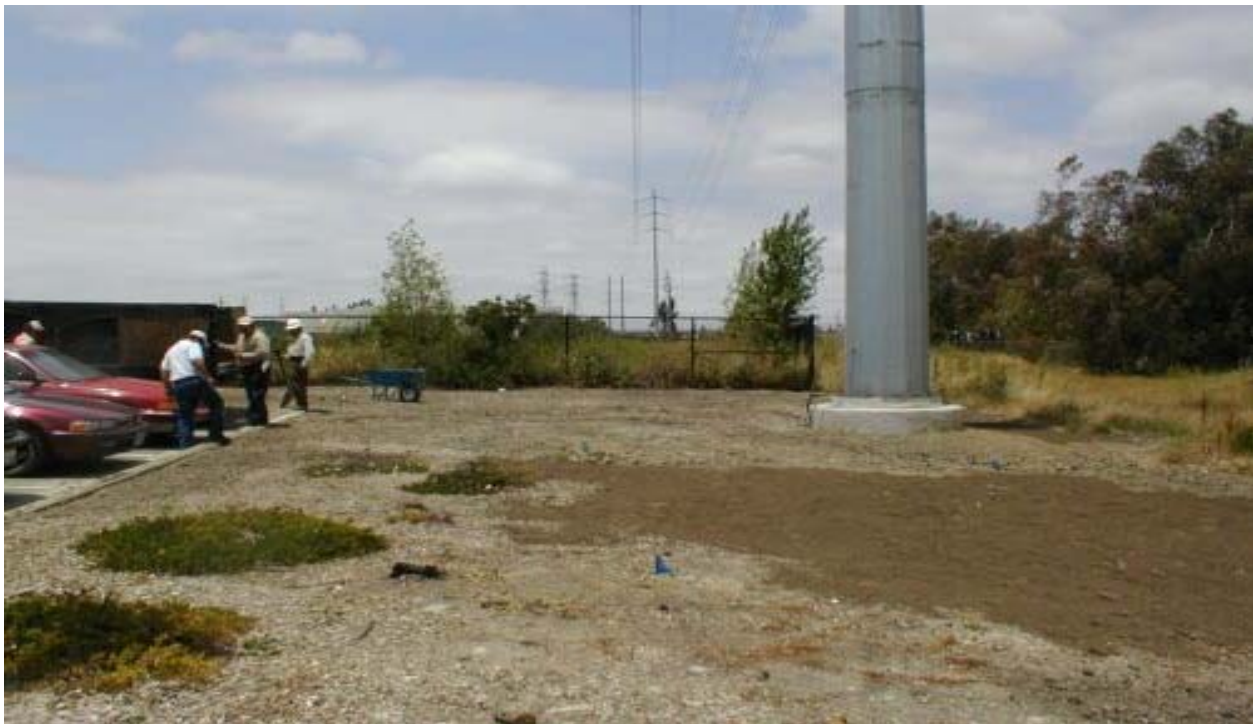
Figure 2 Landscaping Work at Pole #3 June 11, 2003
