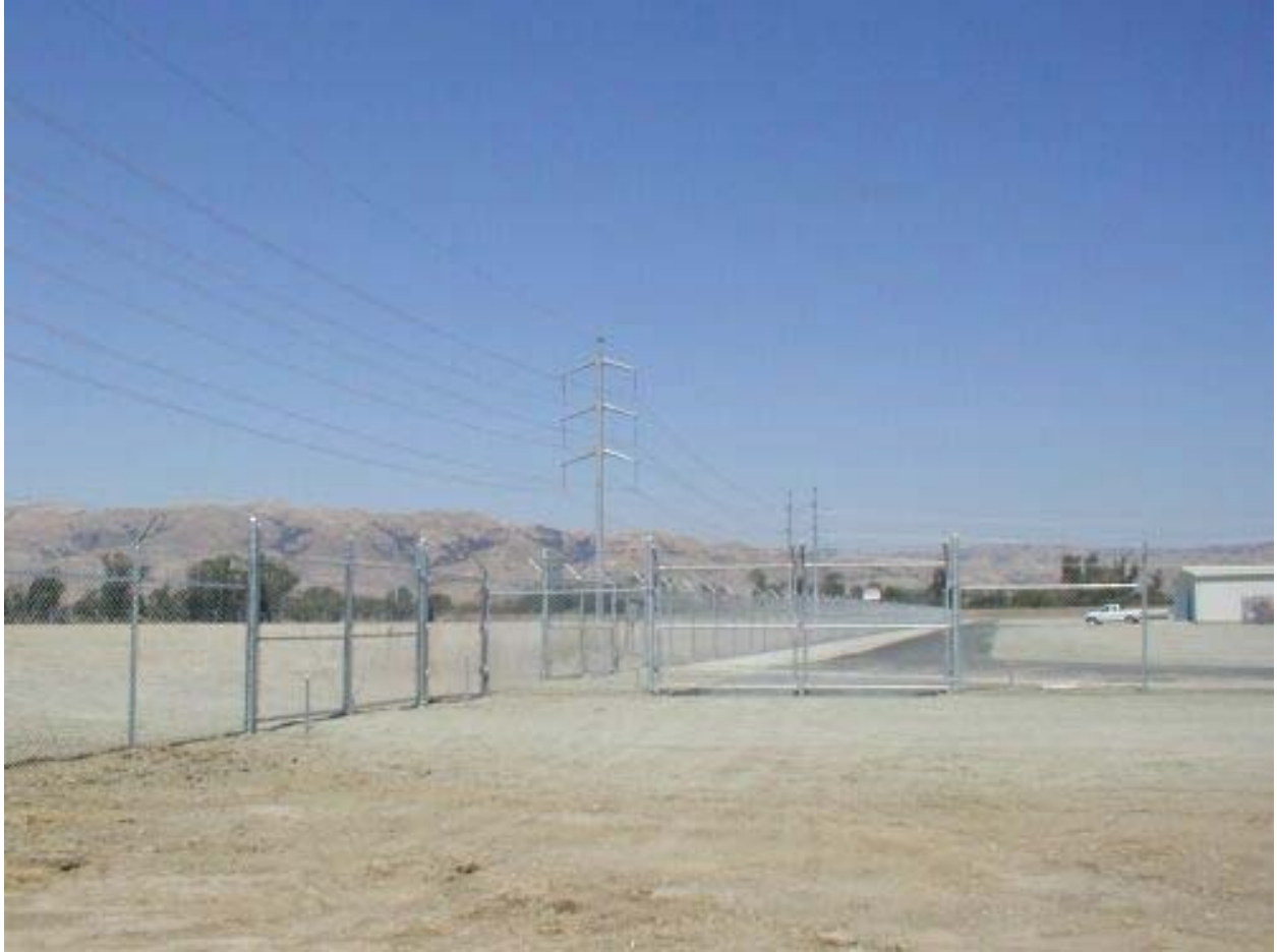
Figure 2 New Fence around North Side of Los Esteros Substation Property June 27, 2003
