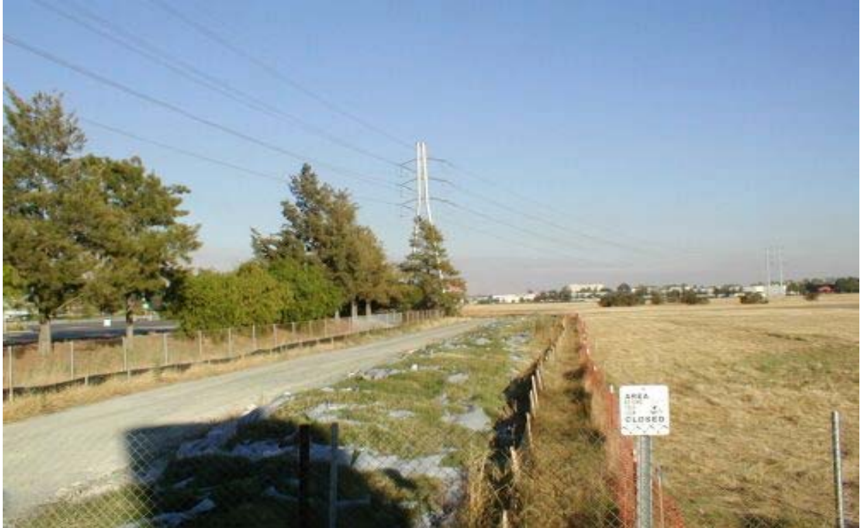
Figure 1 Access Road to Structure #5 on the Catellus Property July 8, 2003
