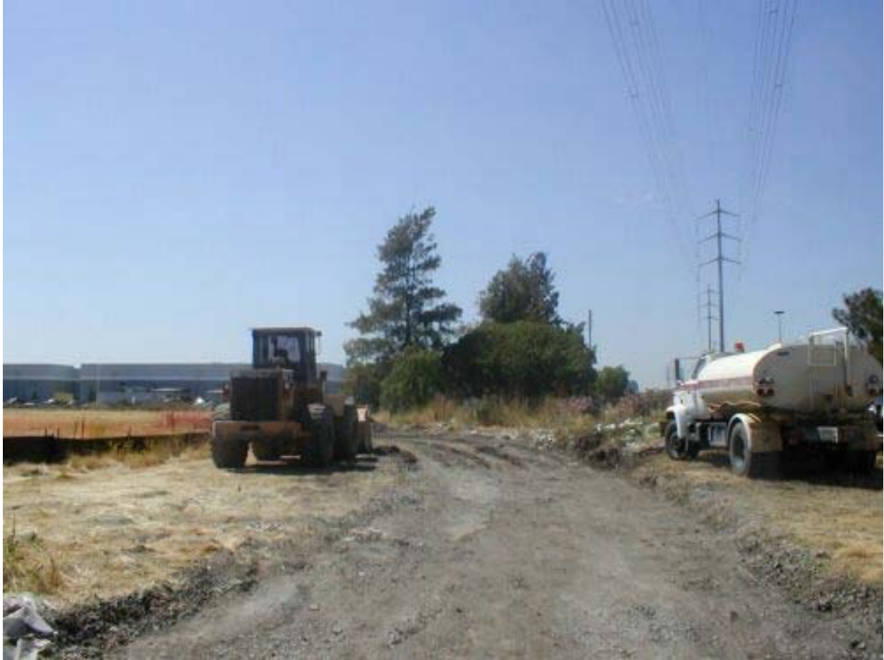
Figure 1 Appian Engineering Crews Removing the Access Road to Pole #5 July 17, 2003
