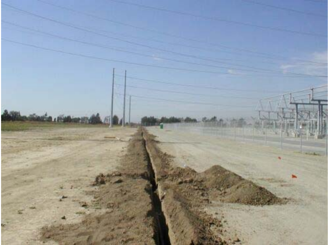
Figure 2 New Water Line Installation for Landscaping July 17, 2003
