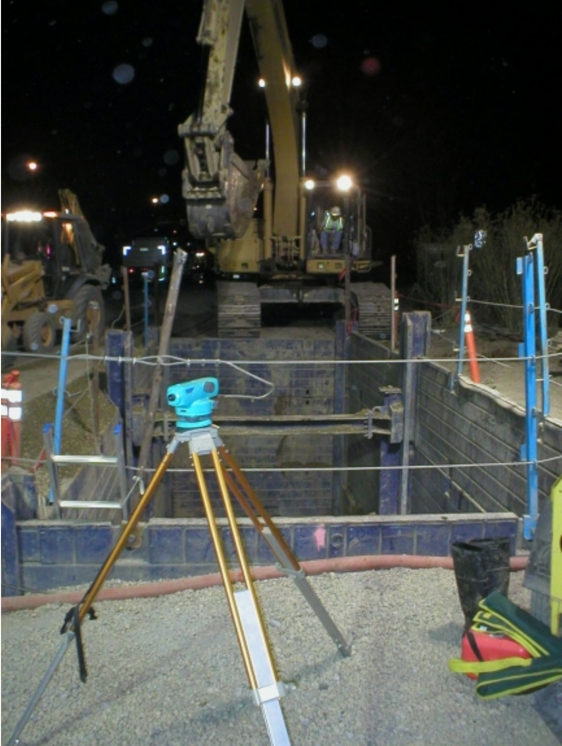
Figure 1: USD Lagoon #4 right line bore entry pit excavation.
