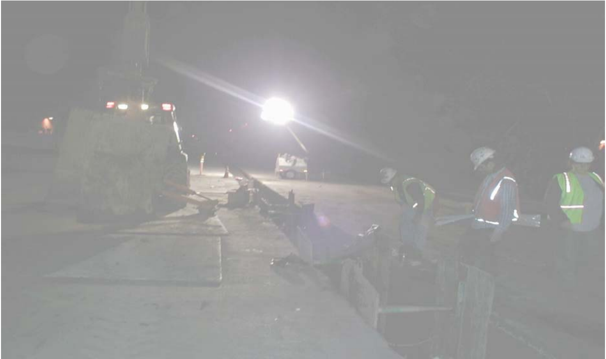
Figure 4 Trenching Work Behind Business Park November 13, 2002
