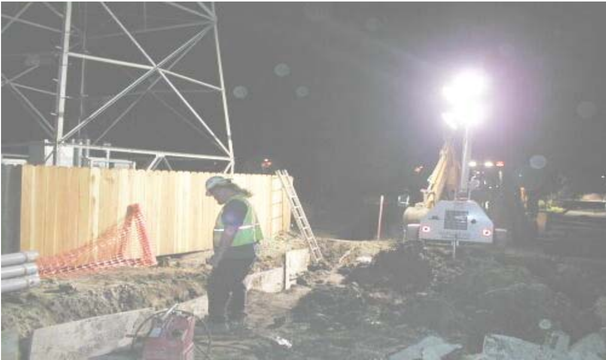
Figure 3 Trenching Work on the Pinole Property South of Vaults #9 November 13, 2002
