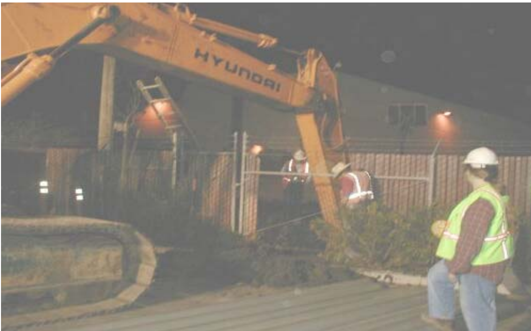
Figure 2 Trenching Activities at Approximately Station 131+00 on the Left Line November 19, 2002
