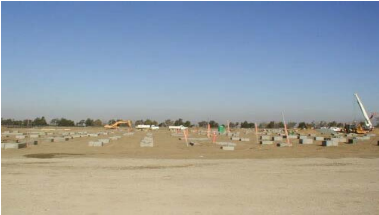
Figure 3 Foundation Work at the Los Esteros Substation November 27, 2002
