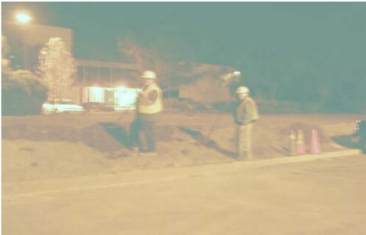
Figure 4 Crews re-contouring berm on Mervyn's Property December 12, 2002
