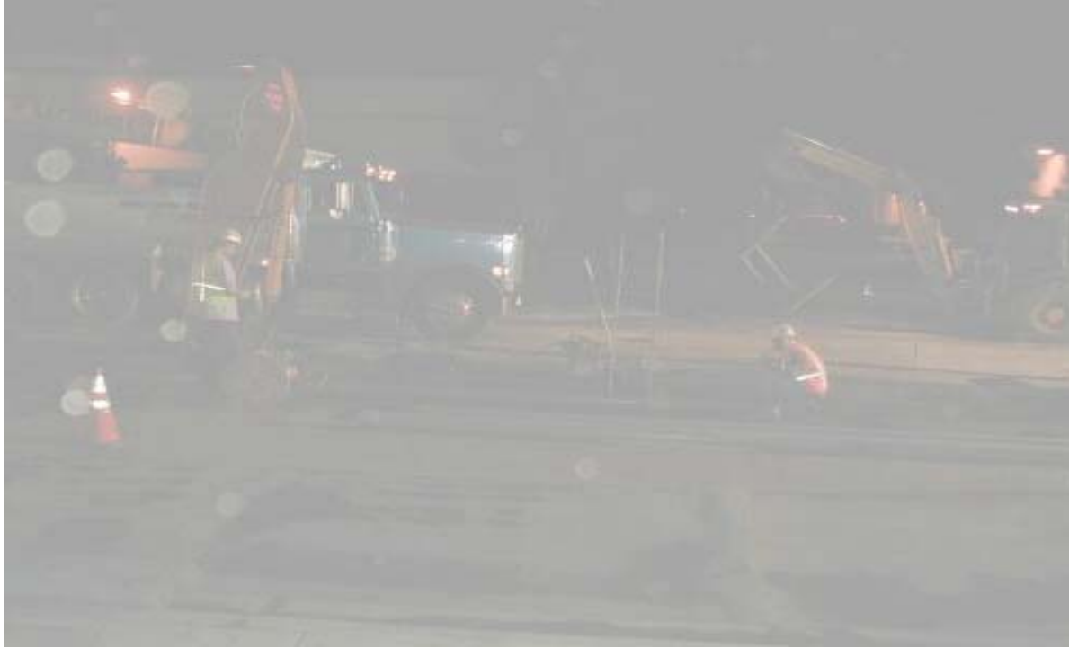
Figure 1 Trenching Activities at South End of Route December 10, 2002
