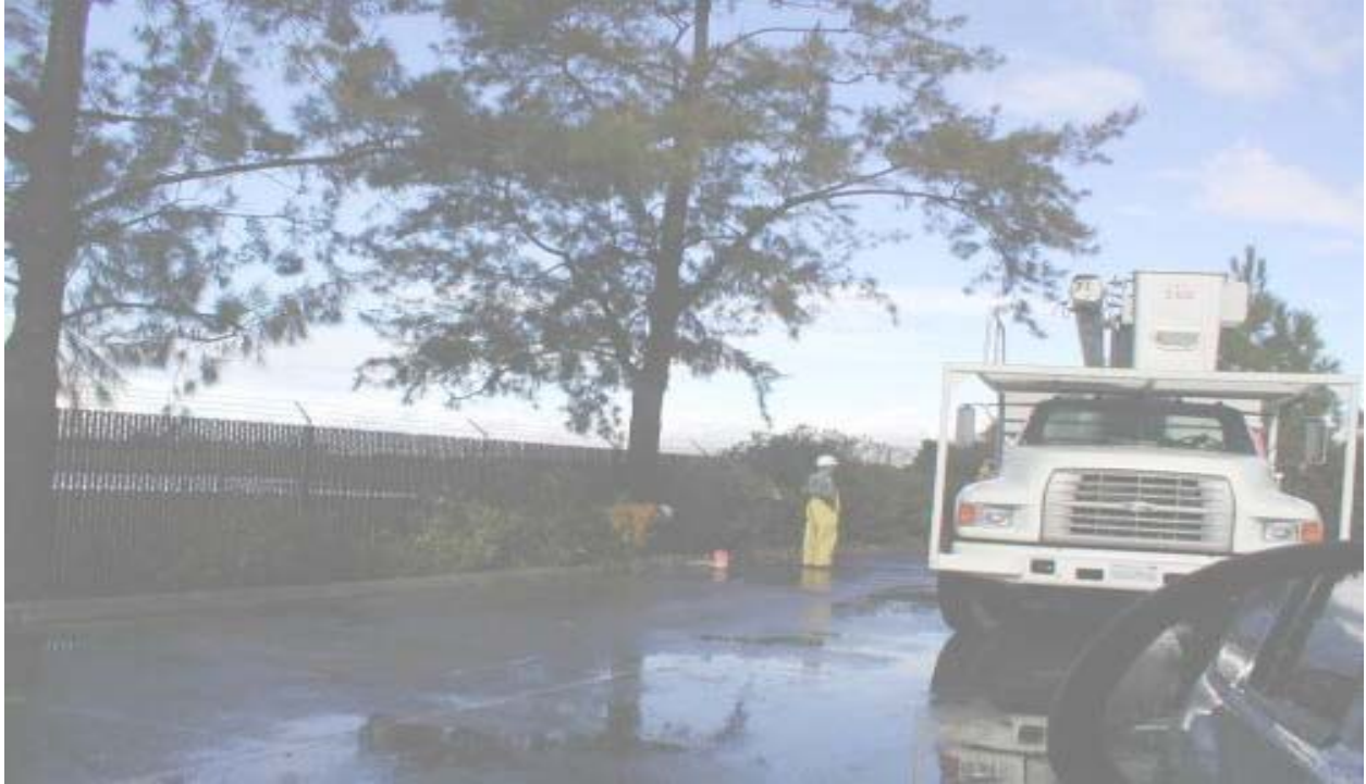
Figure 1 Tree Cutting Activities between Pole Foundations #6 and #9 December 17, 2002
