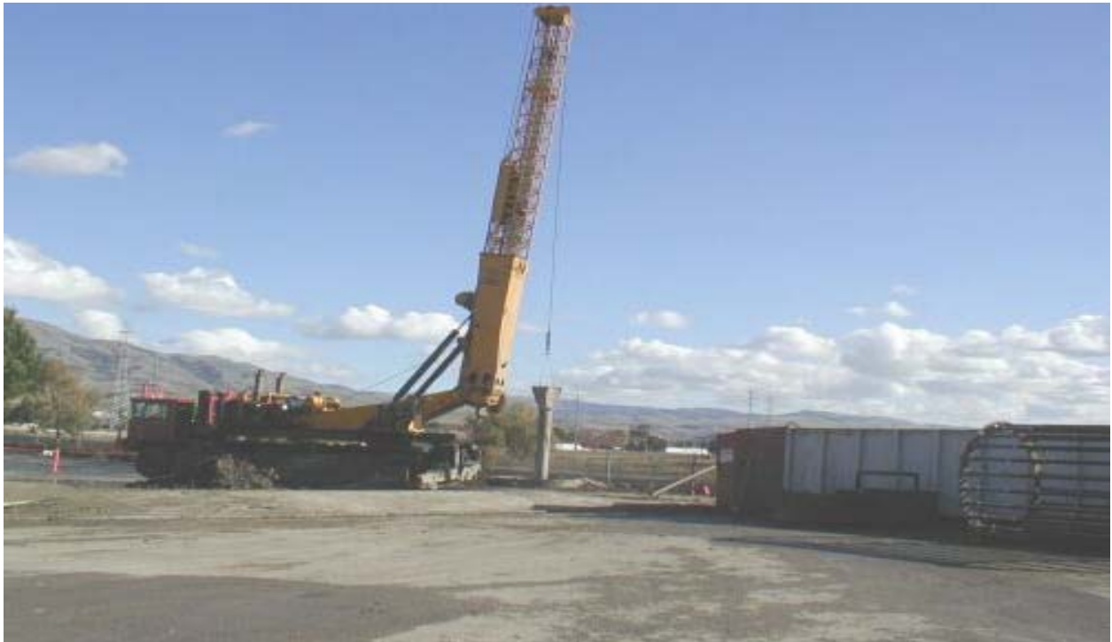
Figure 4 Crews Pouring Pole Foundation 10 L December 18, 2002
