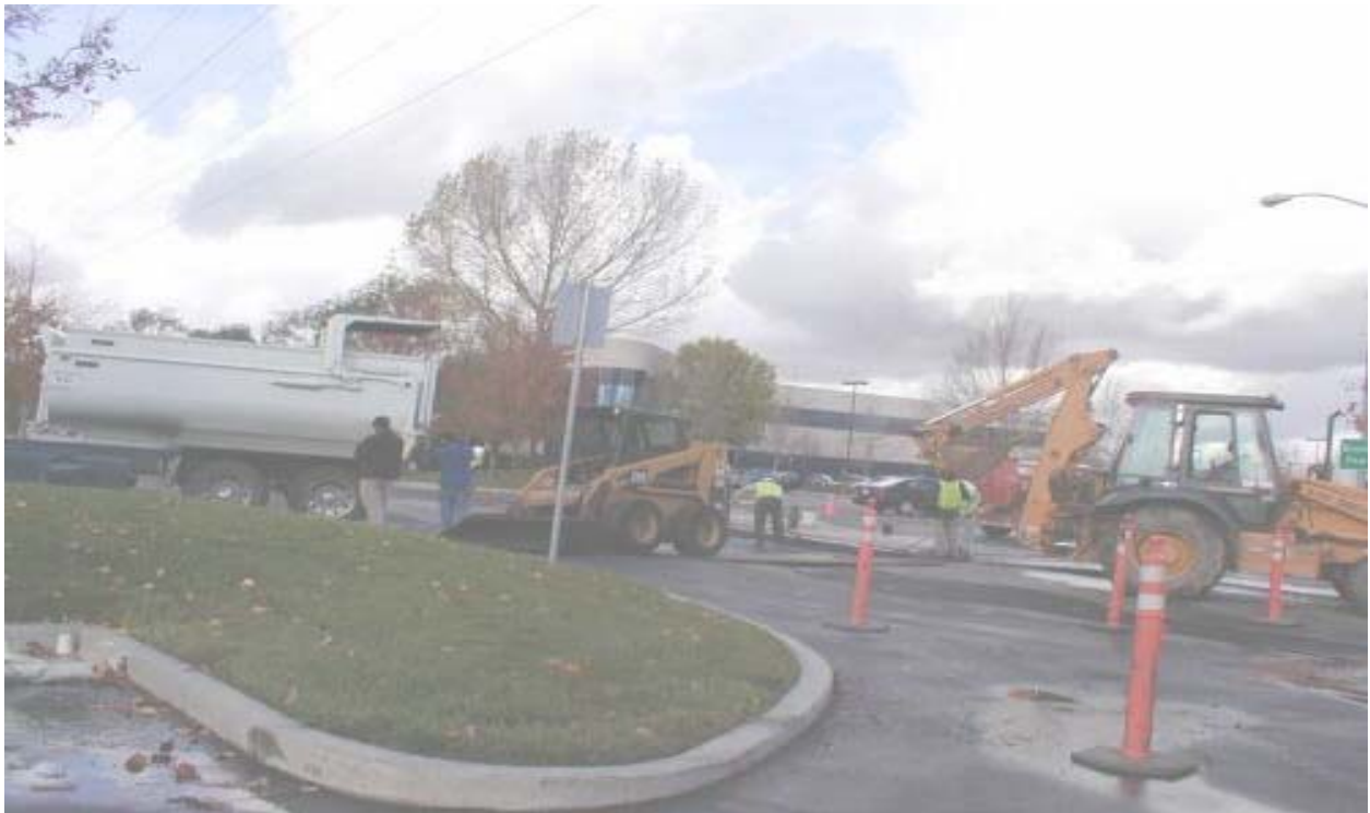
Figure 2 Crews Paving Across Gateway Boulevard December 17, 2002
