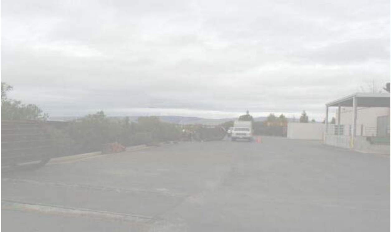
Figure 1 Tree Cutting Service Removing Stumps between Pole Foundations #8 and #9 December 27, 2002
