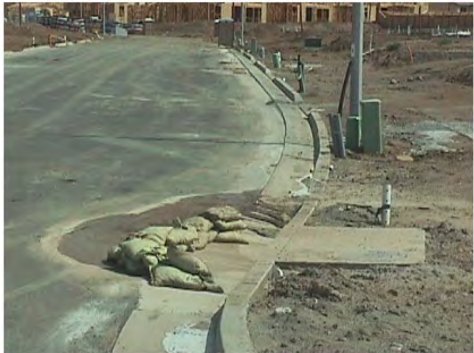
Gravel bag inlet protection.
