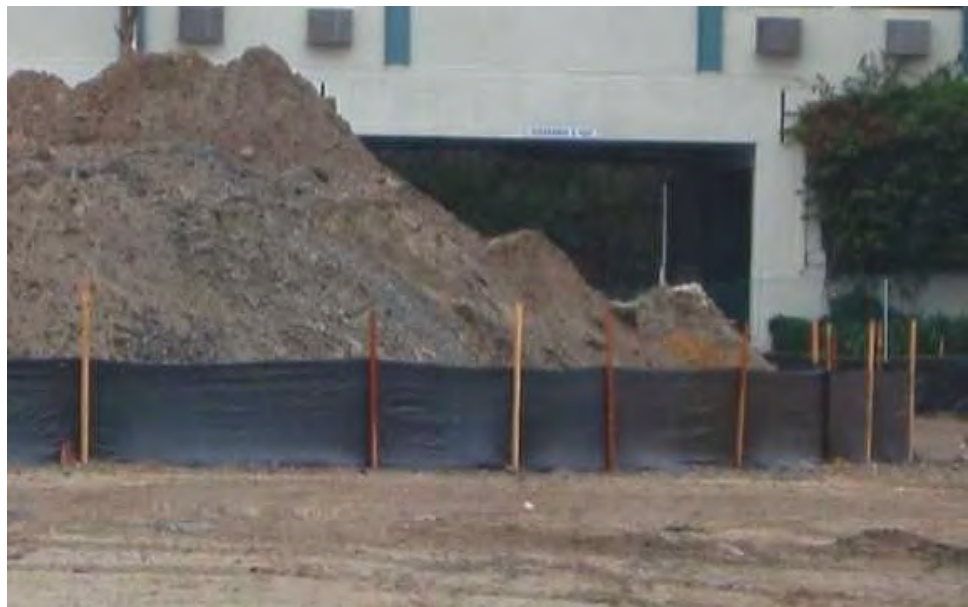
Silt fence used for stockpile perimeter control.
