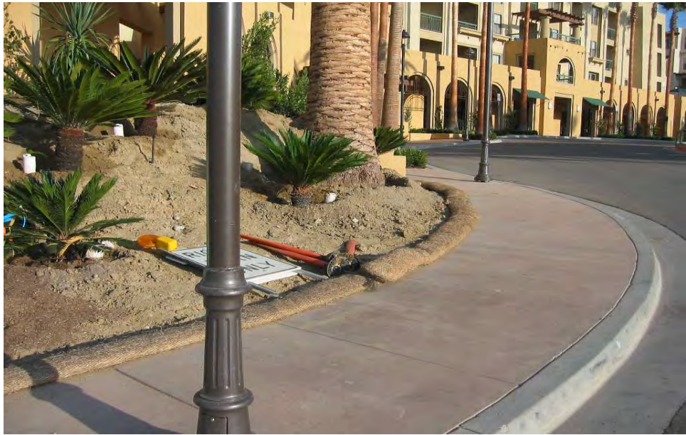
Fiber rolls as perimeter control
