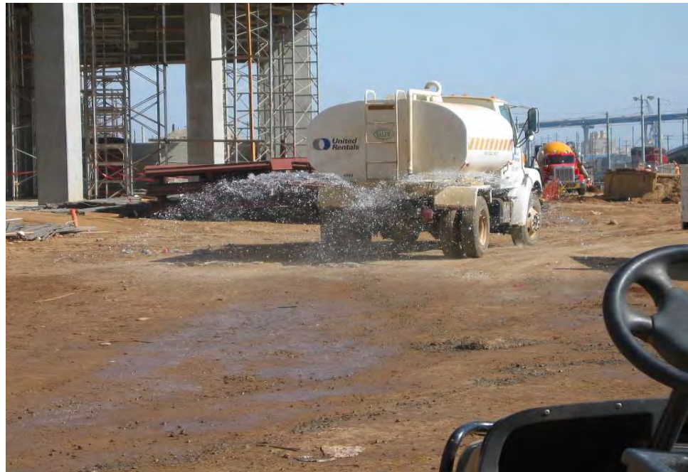
Water being applied for dust control.
