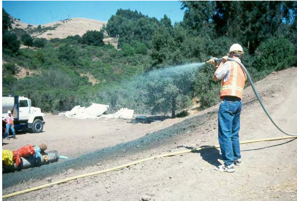
Applying hydroseed.
