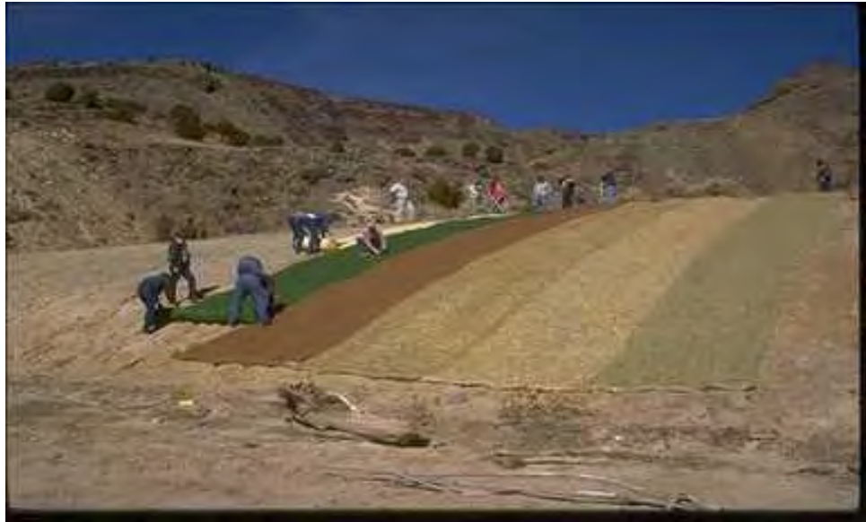
Several types of Erosion Control Blankets.
