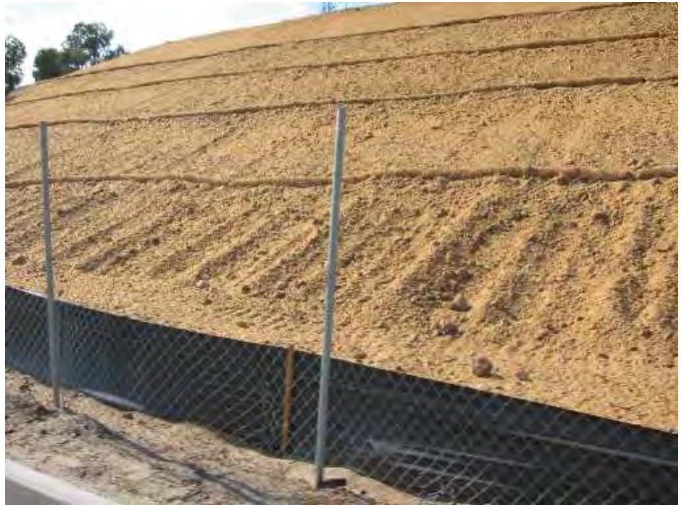
Silt fence installed at the toe of an erodible slope. Note use is combined with fiber rolls and serves as perimeter control.
