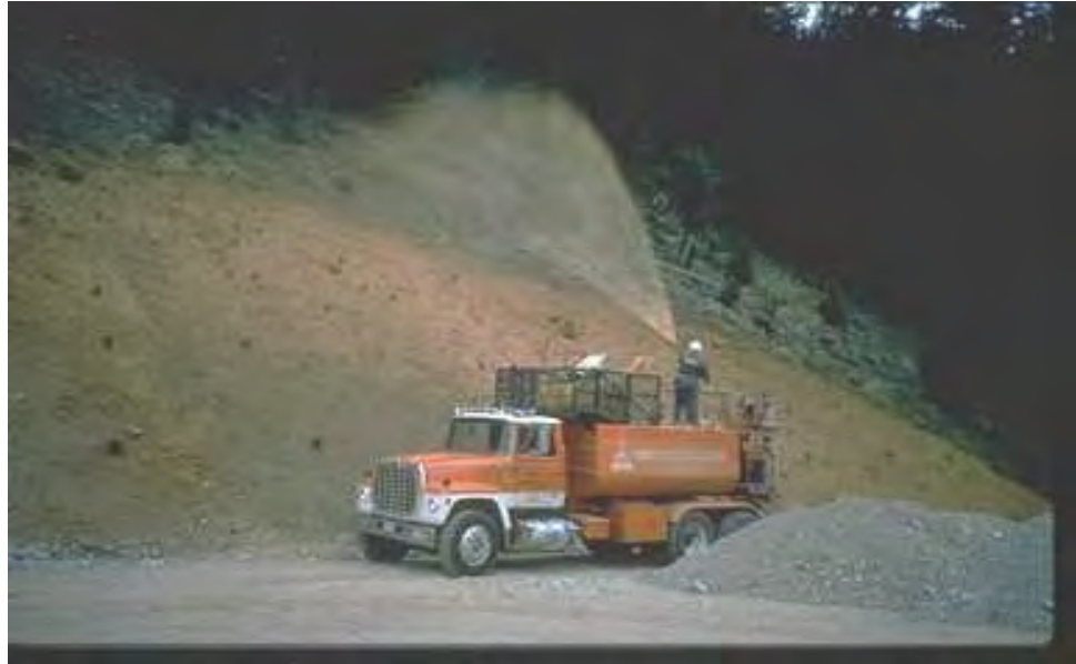
Applying hydraulic mulch.
