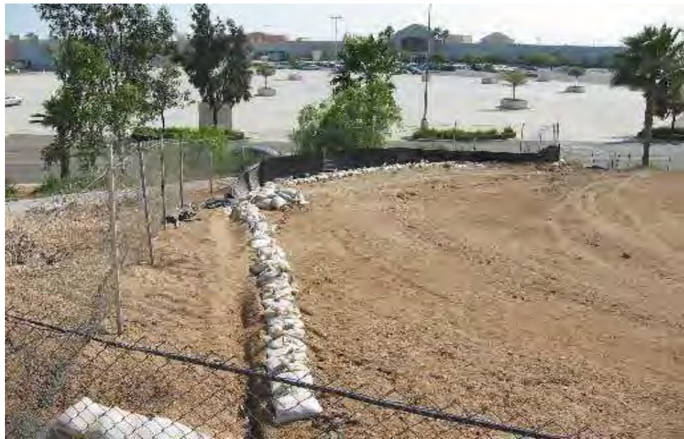
Gravel bags used as perimeter control.
