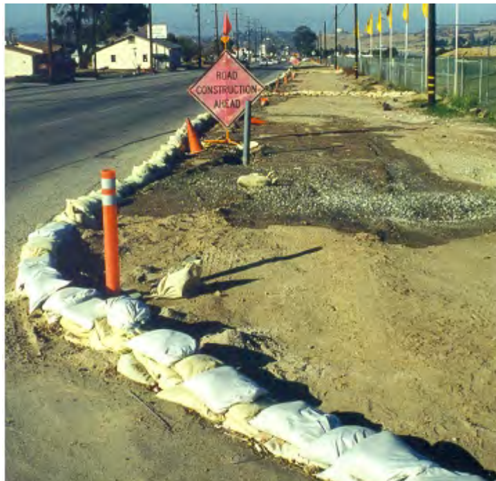
Sand bags used as perimeter control.
