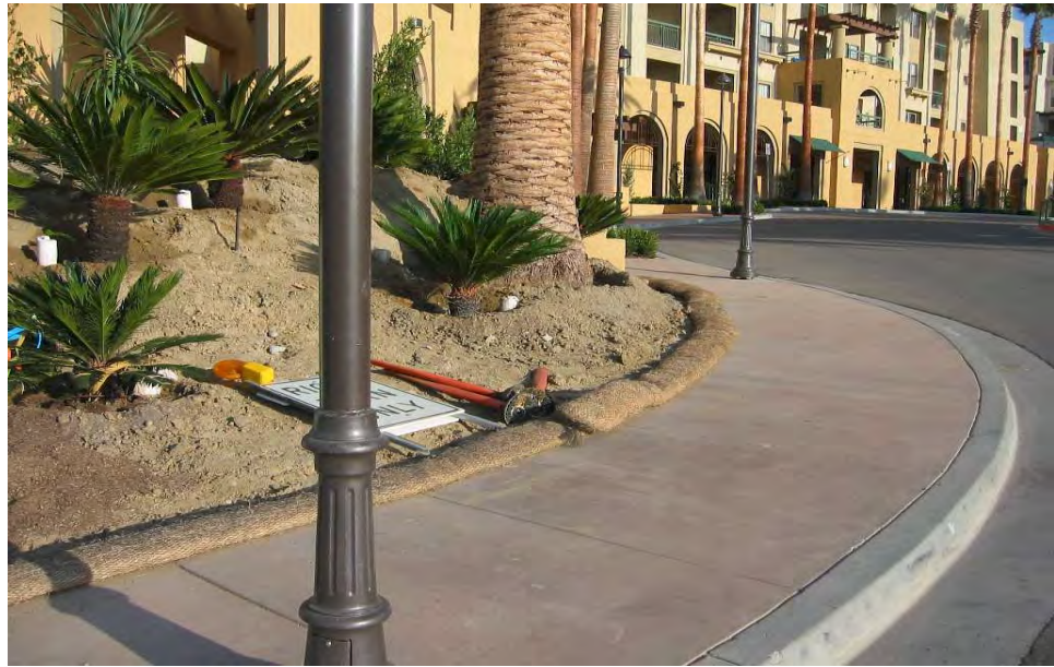
Fiber rolls as perimeter control
