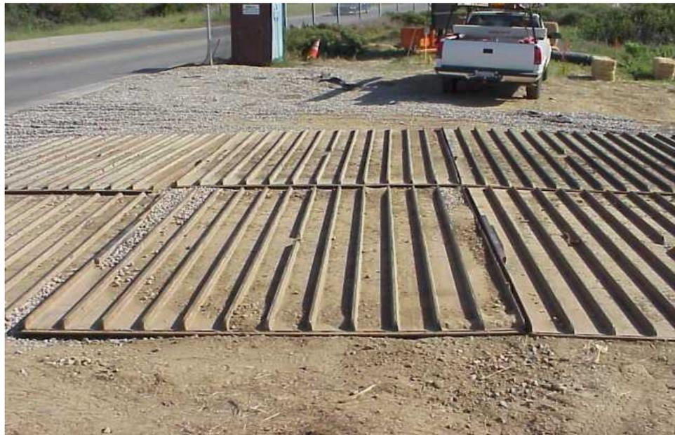
Manufactured metal plates knock dirt off vehicles before exiting a site.
