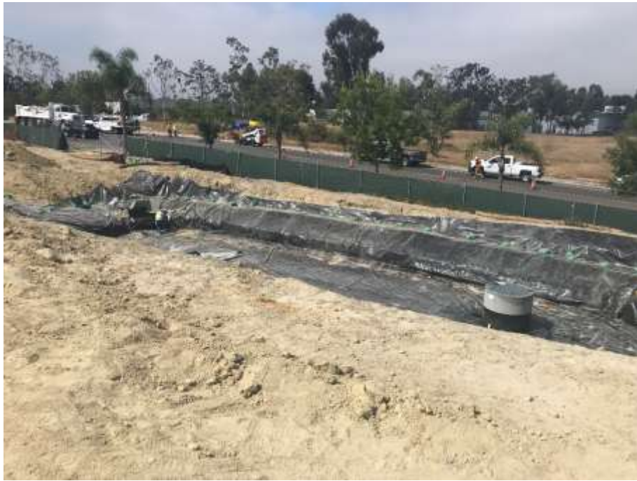
Figure 1 – Installation of substation basin liner looking toward Avenida Del Oro, July 25, 2018.
