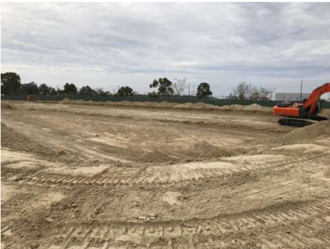
Figure 2A – Progression of Basin construction, March 2018.
