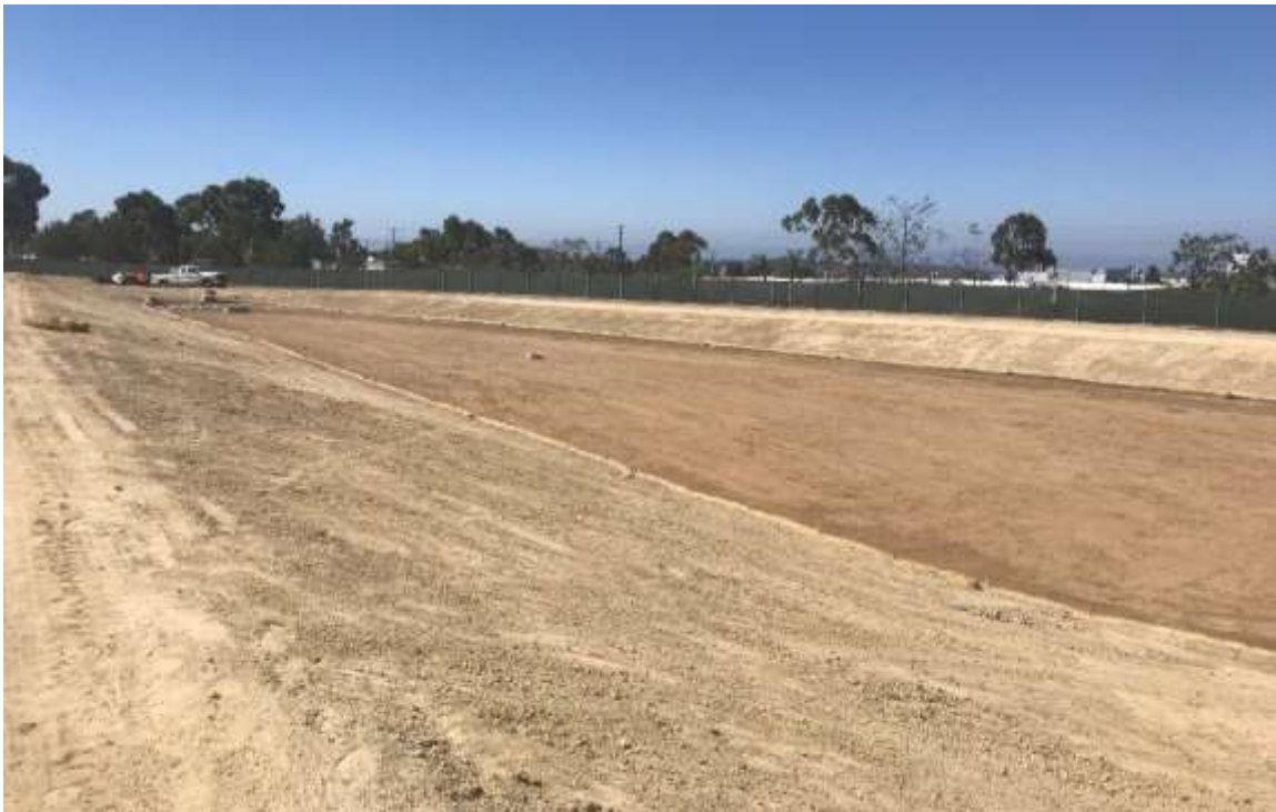
Figure 2C – Progression of Basin construction, October 2018.
