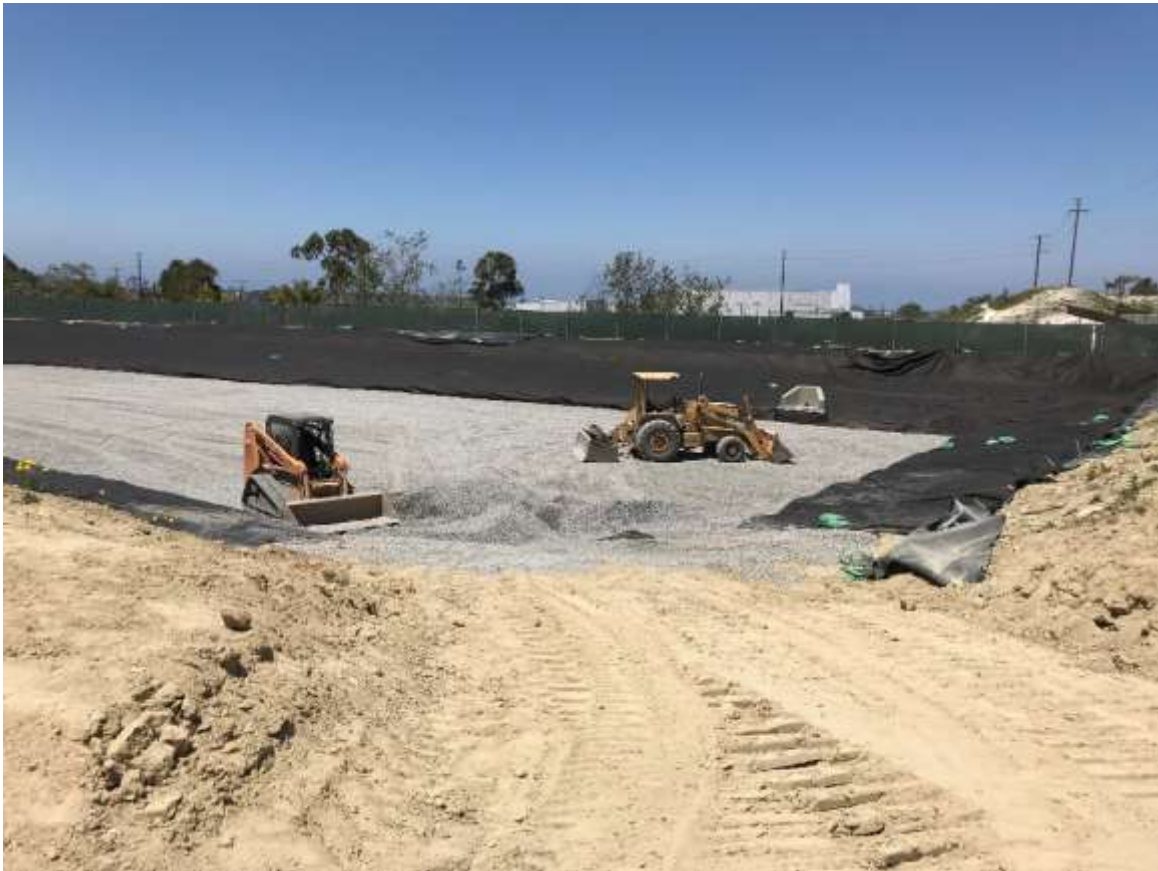
Figure 2B – Progression of Basin construction, June 2018.
