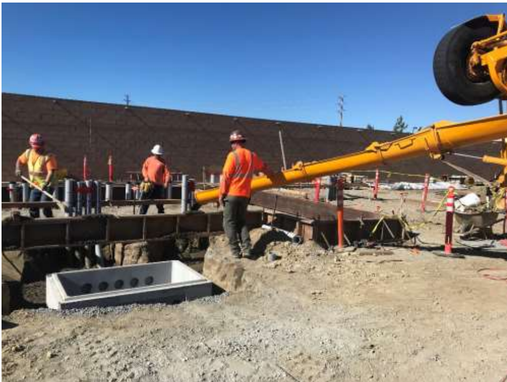
Figure 2 – Form placement and foundation pouring inside the substation, January 23, 2019.
