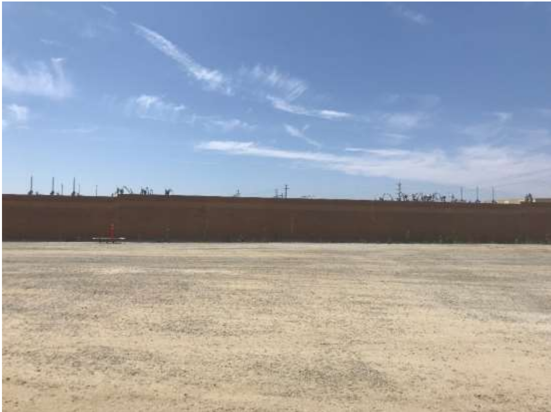
Figure 2 – Class 2 base surrounding the low-profile Ocean Ranch Substation, July 23, 2019.
