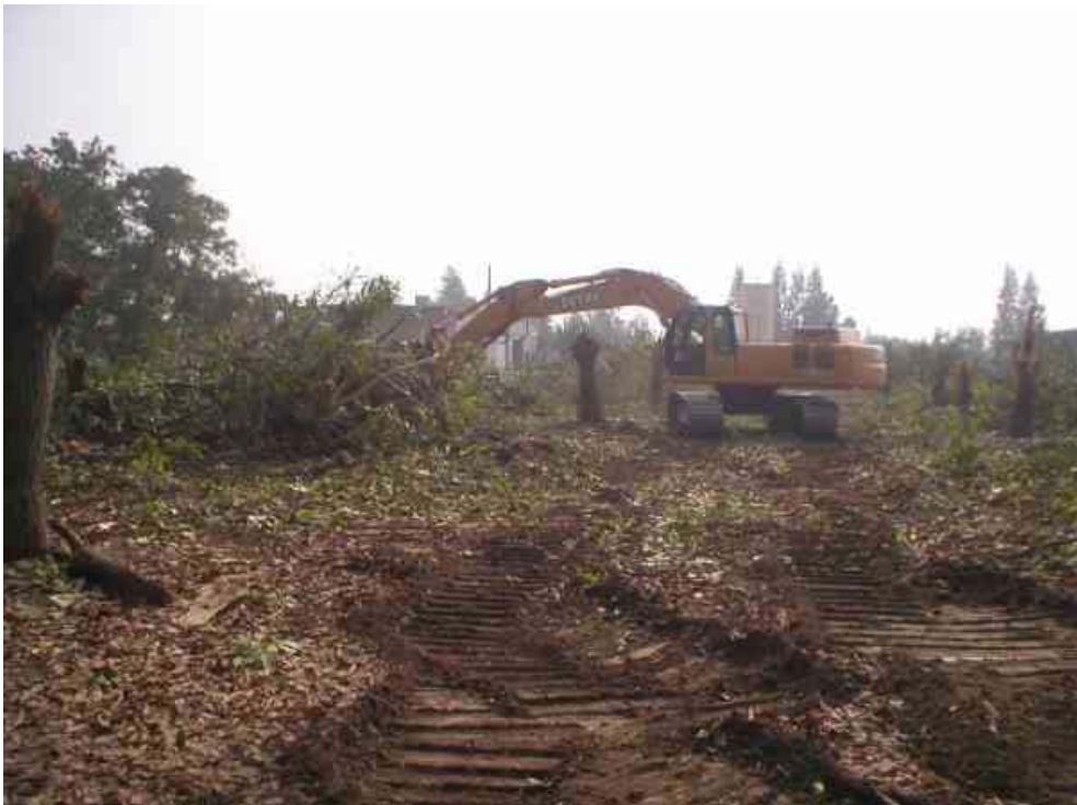
Figure 2 – Crews putting up the tree roots with an excavator, November 1, 2007.
