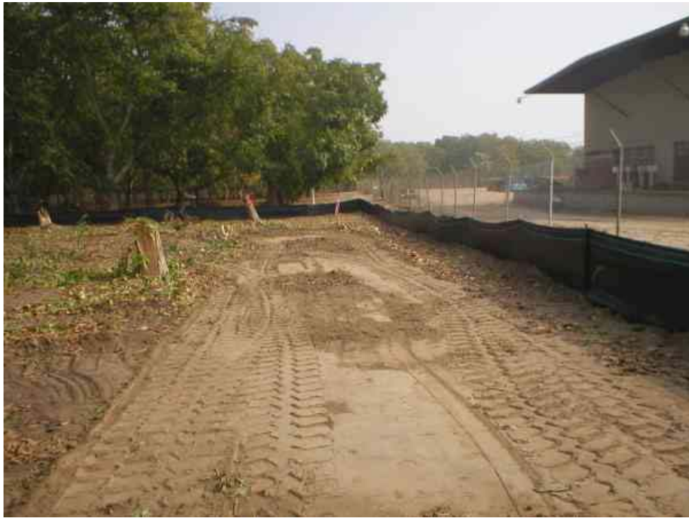
Figure 5 – Sediment fence installation around the future substation site, November 1, 2007.
