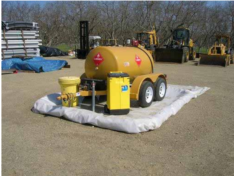
Figure 1: Prior to February 10 th , 2008, the laydown yard had been prepared and stacked with materials for the civil phase of the Project.
