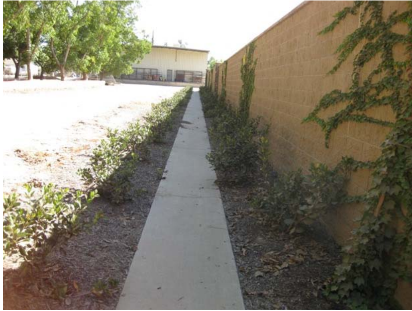
Figure 1: The shallow V-ditch outside the station on the eastern side is now surrounded by well-tended landscaping, including the climbing vine. The photograph faces southward.
