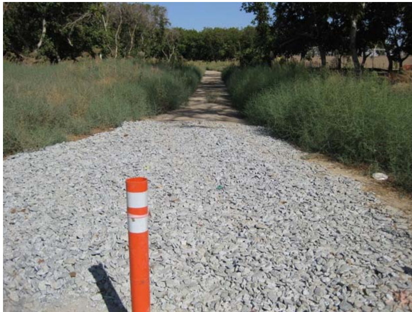
Figure 4: The access road from Mooney Street (behind the photograph) remains unfinished. The western end of the road is gravelled. The road is used as access to the station, but is mostly clogged with Russian thistle. Apparently no work has been done on this road or the adjacent retention basins since August 2008. The substation lies to the right in the distance. The photograph faces eastward.
