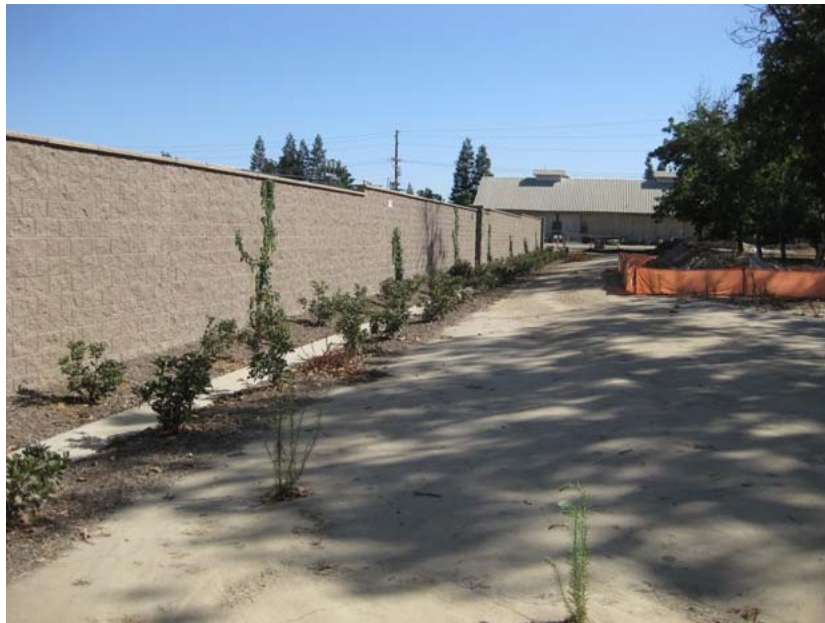
Figure 3: The perimeter of the western side of the station contains well-tended landscaping on both sides of the shallow V-ditch. A secured pile of material remains from the earlier landscaping work. The photograph faces southward.
