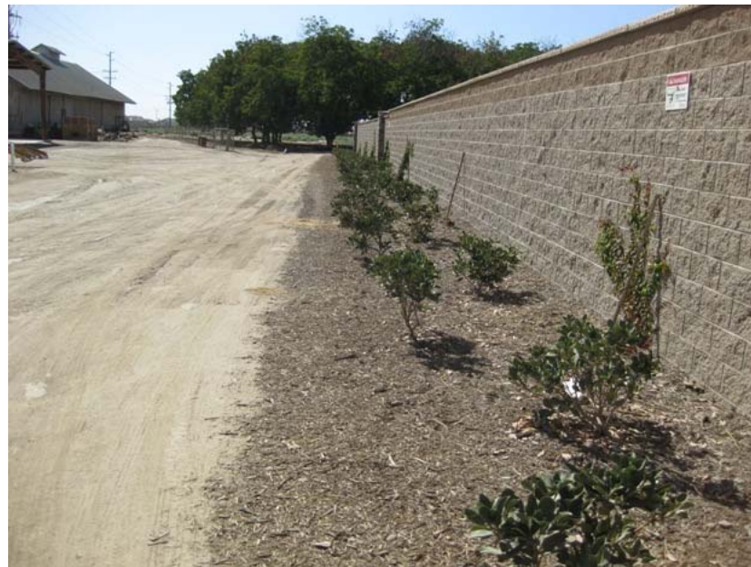
Figure 2: The perimeter of the southern side of the station contains landscaping, but by design, no drainage ditch. The photograph faces westward.
