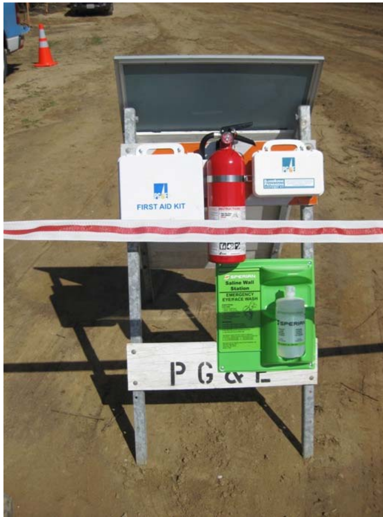
Figure 4: Emergency first aid and fire extinguisher kits are clearly visible and accessible at the entrance to the work area.
