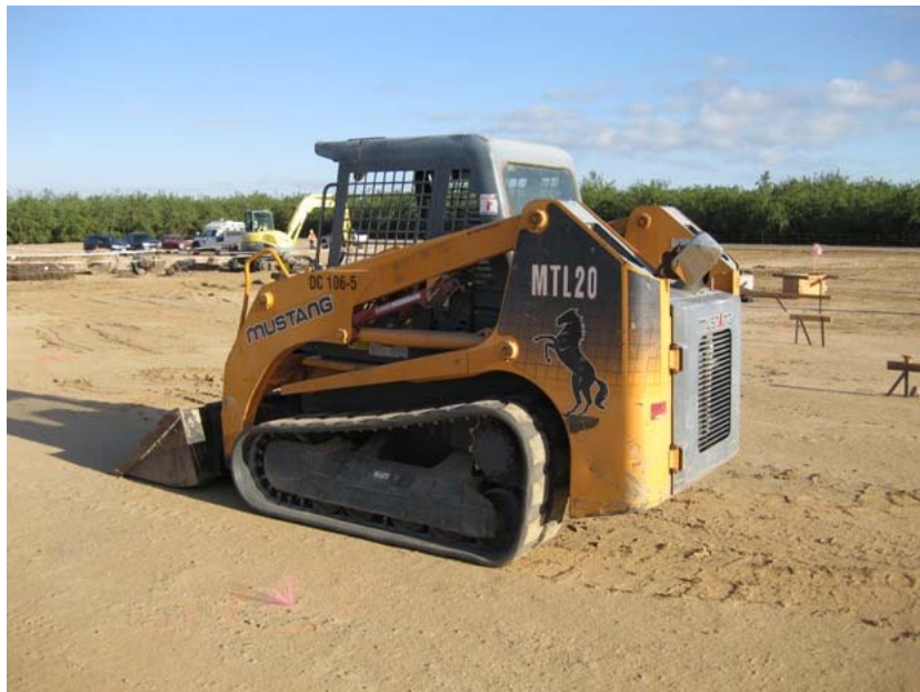
Figure 6: This piece of equipment initially arrived on site with caked dirt on its undercarriage. The contractor was asked to take it off site and get it cleaned. The photograph faces westward.
