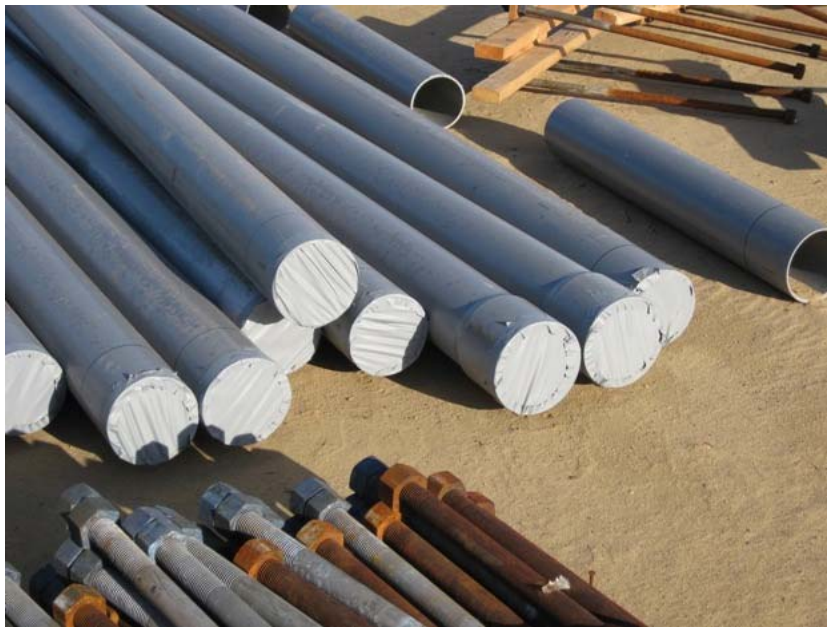
Figure 4: The pipe stored on site with diameters four inches and greater and more than four feet in length are covered to discourage usage by animals.
