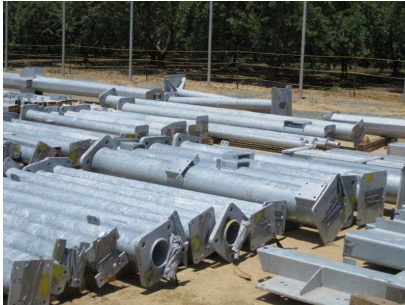
Figure 9: This batch of tower parts was sealed with tape upon delivery on site. The combination of poor quality tape, improper installation, and temperature changes caused some of the seals to fail. The contractor was directed to use different material to seal the pipes properly. The photograph was taken in the laydown yard in the western portion of the site, and faces northwestward.
