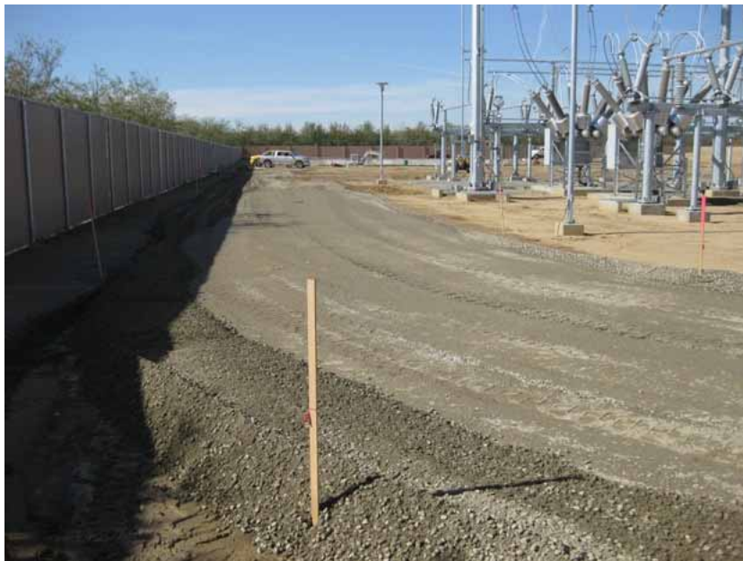
Figure 2: Final grading and placement of road base occurred during the subject period. The photograph faces southward.
