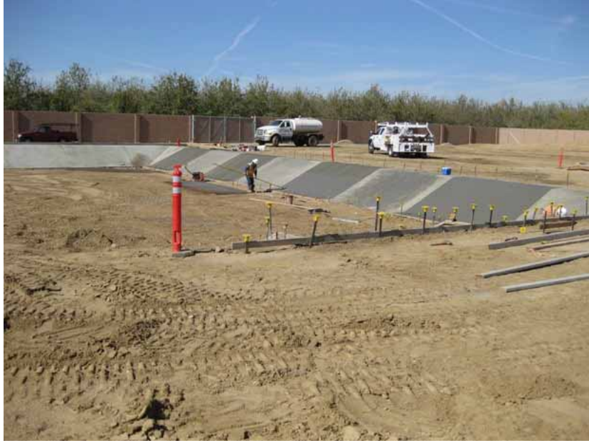
Figure 3: During the subject period, the slopes of the retention basin were lined with concrete and the native material comprising the floor of the basin was graded. The photograph faces northwestward.
