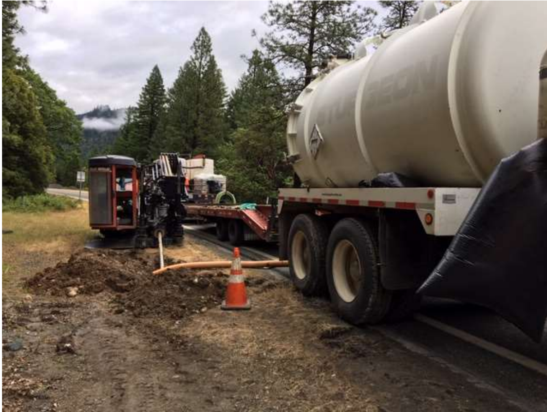
Figure 1 – Crew drilling at MP 24.5 south along Hwy 96 – view north, May 22, 2019.
