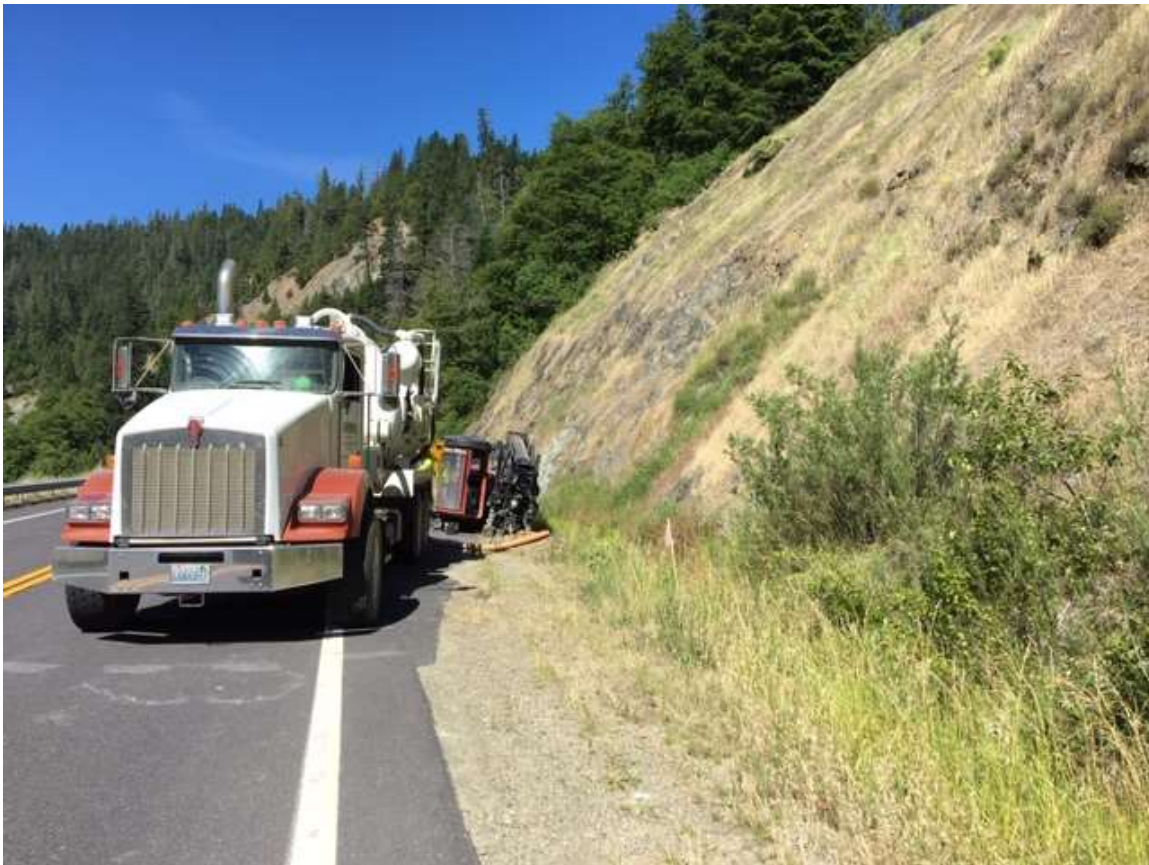
Figure 4 – Crew Drilling northeast at MP 29.16 – view southwest, June 5, 2019.
