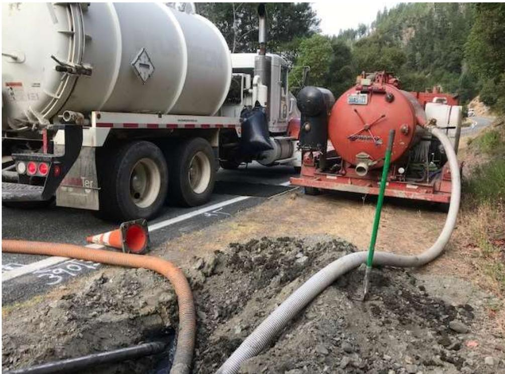
Figure 2 – Absorbent pad placed under vac-truck as precaution to avoid spills – view north, August 7, 2019.
