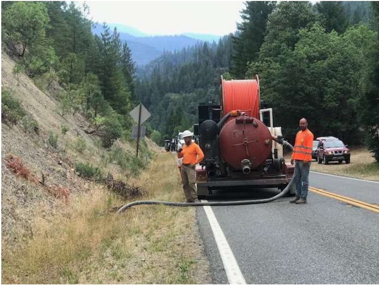
Figure 3 – Vac truck placed in position to clean up frac-out at MP 29.8, view north, August 28, 2019.
