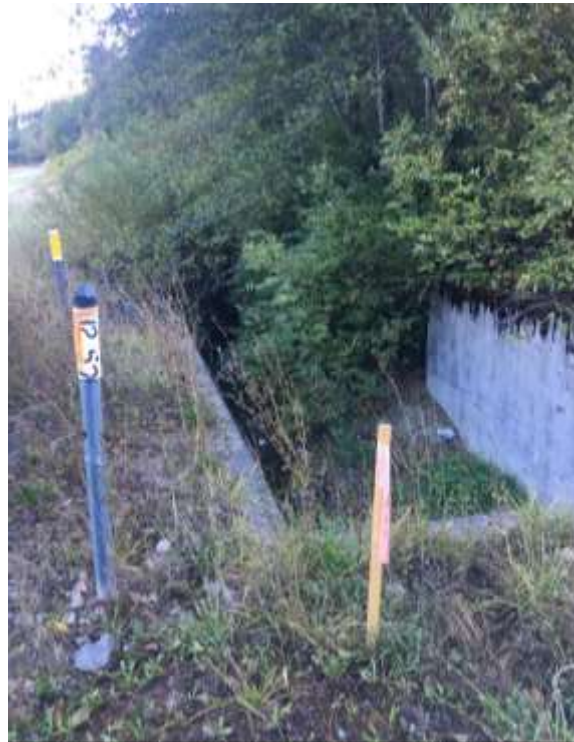
Figure 4 – Staking and flagging of wet culvert, MP 12.59. September 25, 2019.
