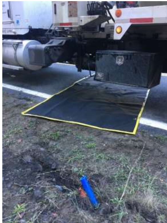
Figure 2 – Absorbent placed under equipment to avoid leaks – September 25, 2019.
