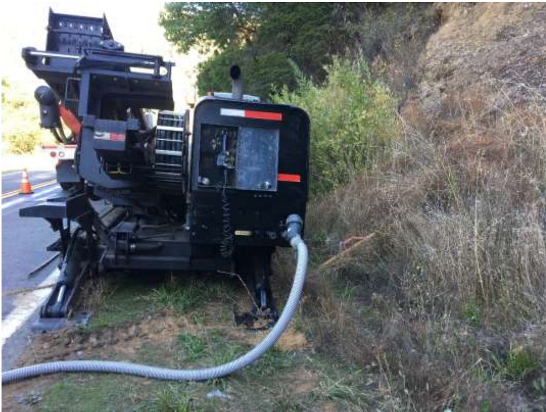
Figure 4 – HDD equipment staged near sensitive habitat staking, October 9, 2019
