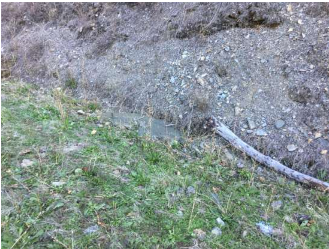
Figure 5 – Frac-out needing clean-up, observed by CPUC EMs, MP 13.30, October 9, 2019.
