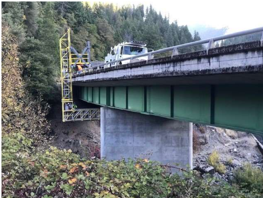
Figure 3 –Bridge handing operations at Clear Creek Bridge – view north, October 9, 2019.
