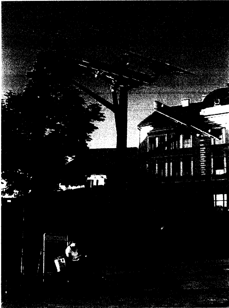
Solar tree in Styria Austria (70 panels on 5 branches, occupying about 1 square foot on the ground)
