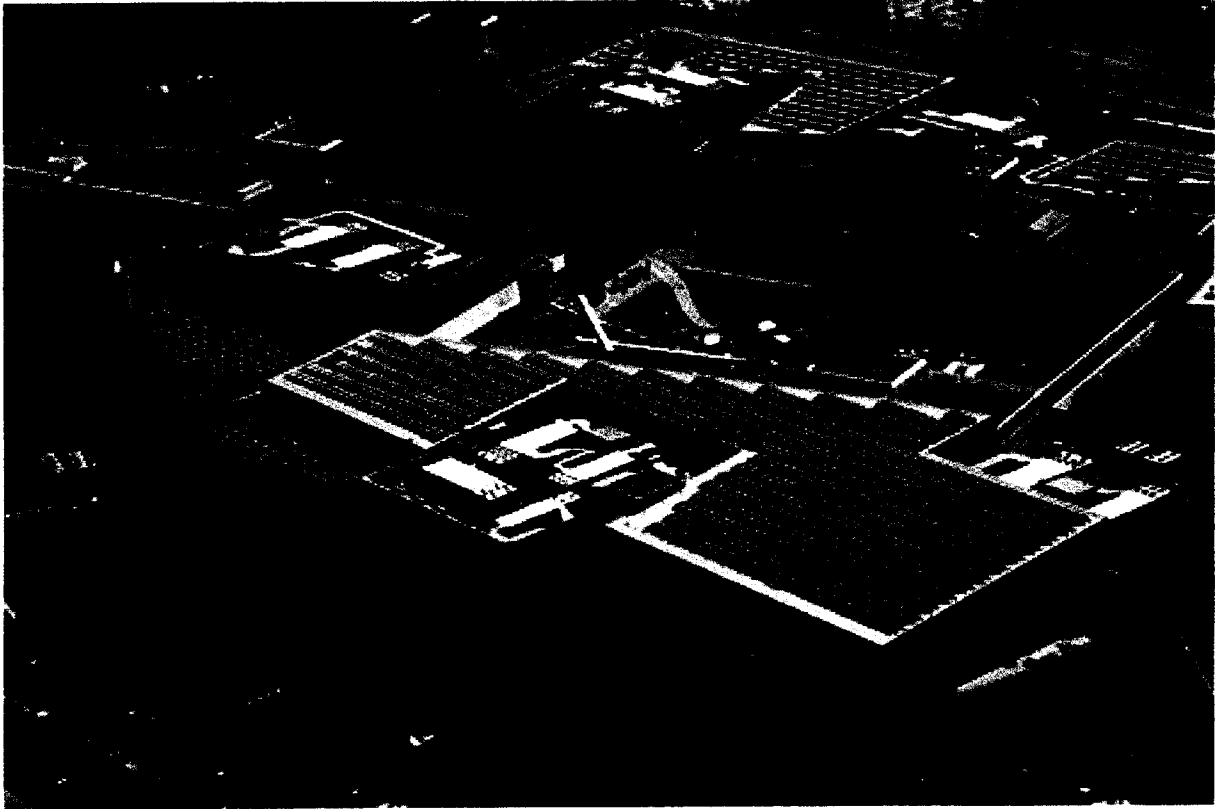
1.6 megawatts from the roof of Google's offices
