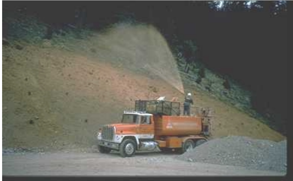
Applying hydraulic mulch.
