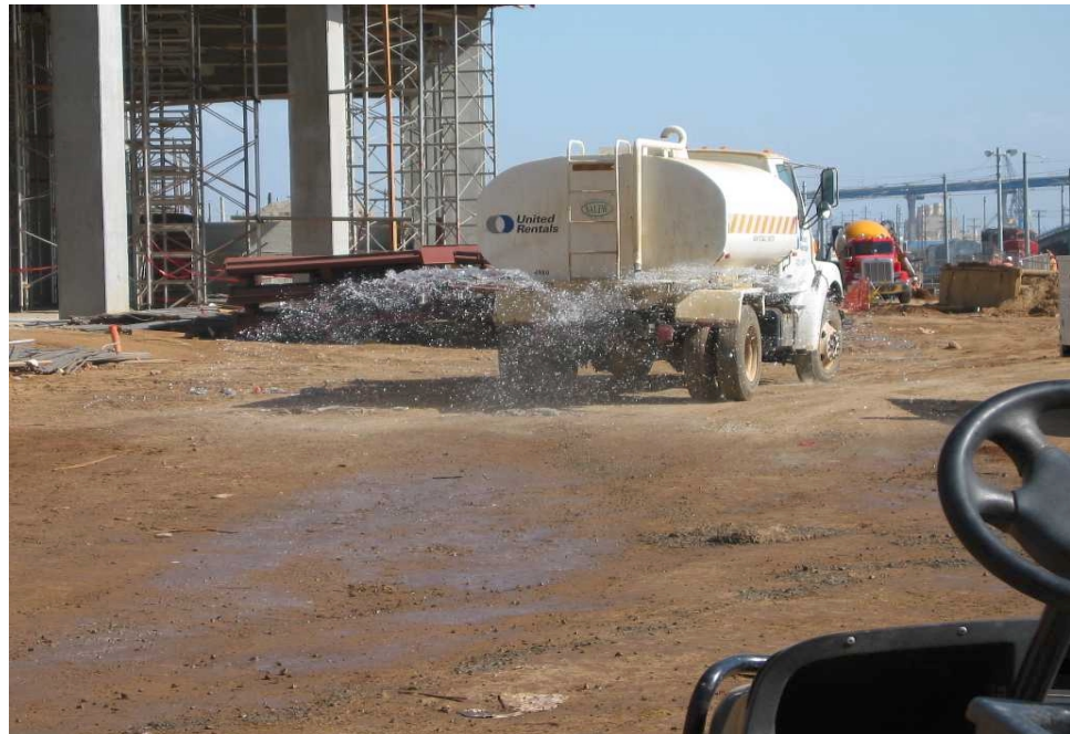
Water being applied for dust control.
