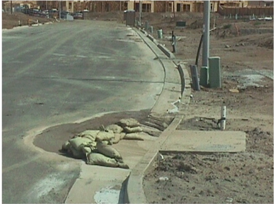
Gravel bag inlet protection.
