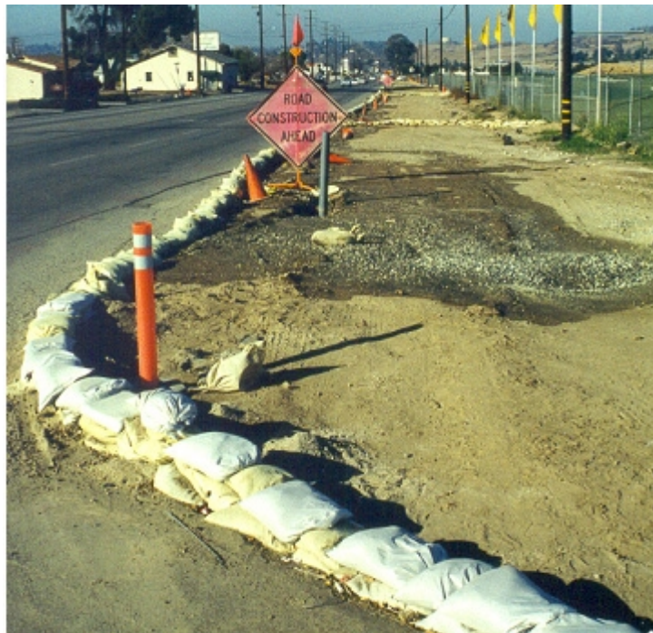
Sand bags used as perimeter control.
