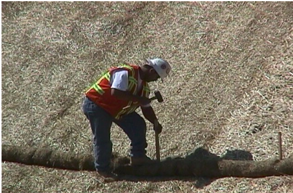
Fiber roll installation on the face of a slope.
