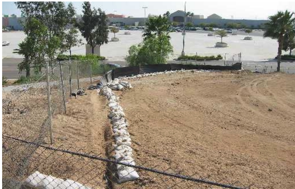
Gravel bags used as perimeter control.
