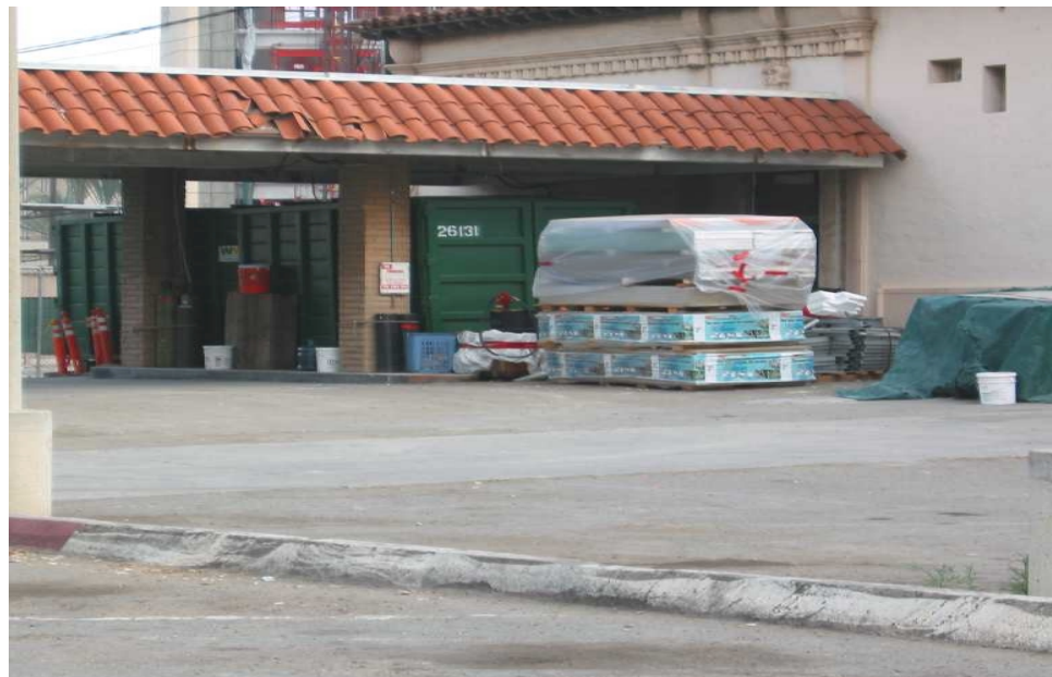
Materials are covered and neatly stored with a curbed area.
