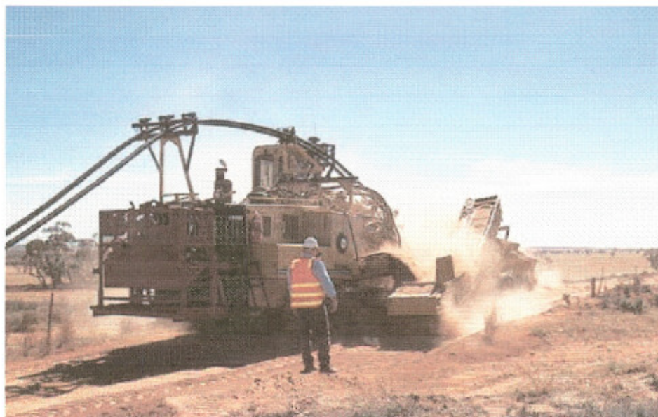
Installation of 110-mile underground DC cable in Australia (Murraylink)
