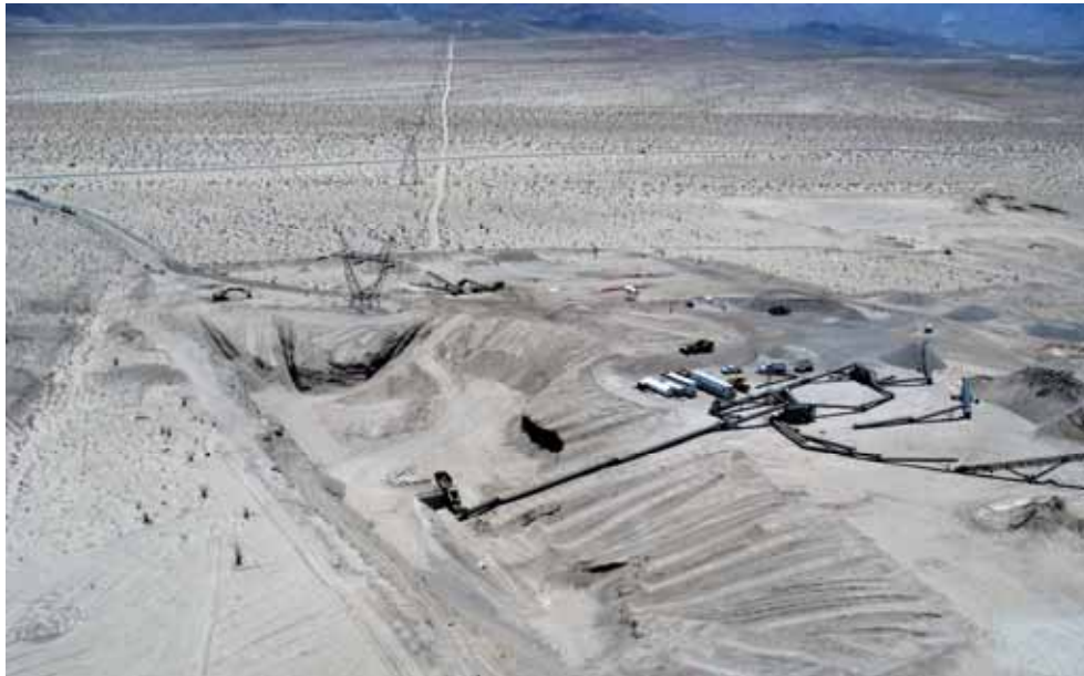
Figure E.1.13-A. SWPL Tower in Mine Area
