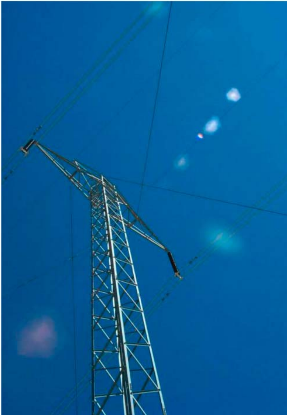
Pacific Intertie 3,100 megawatts, +/-500 kV DC, 1965 LADWP
