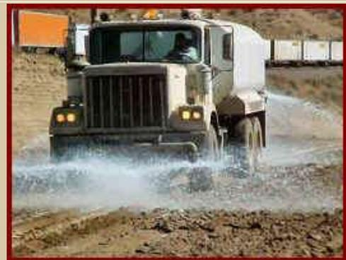
**Simultaneously, the water truck spreads the PX-300/ water mixture over the area undergoing the disc process.**
