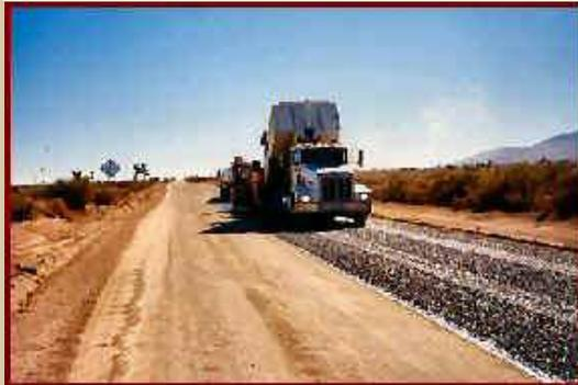
**Chip seal over a PX-300 stabilized road bed provides a simple and durable wear surface for this road in San Bernardino County, California.**
