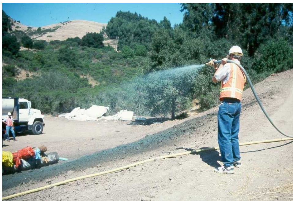
Applying hydroseed.
