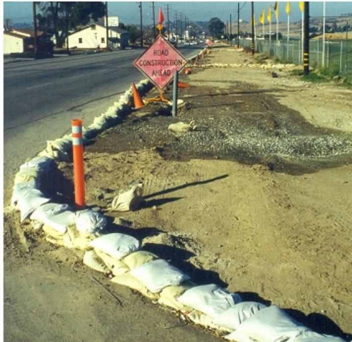
Sand bags used as perimeter control.
