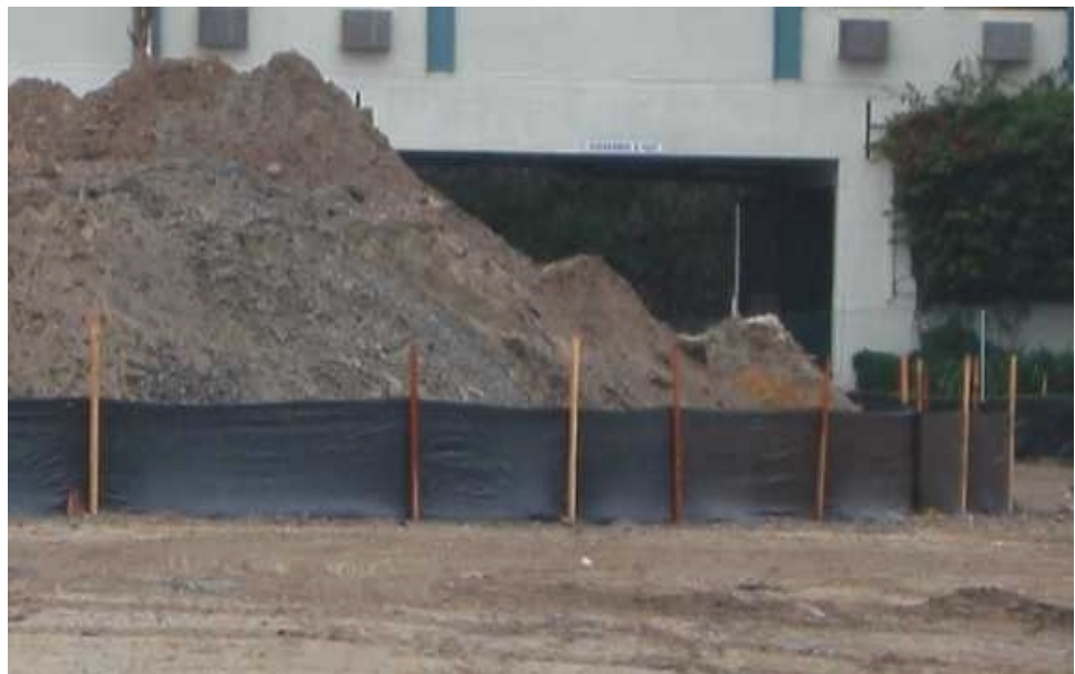
Silt fence used for stockpile perimeter control.
