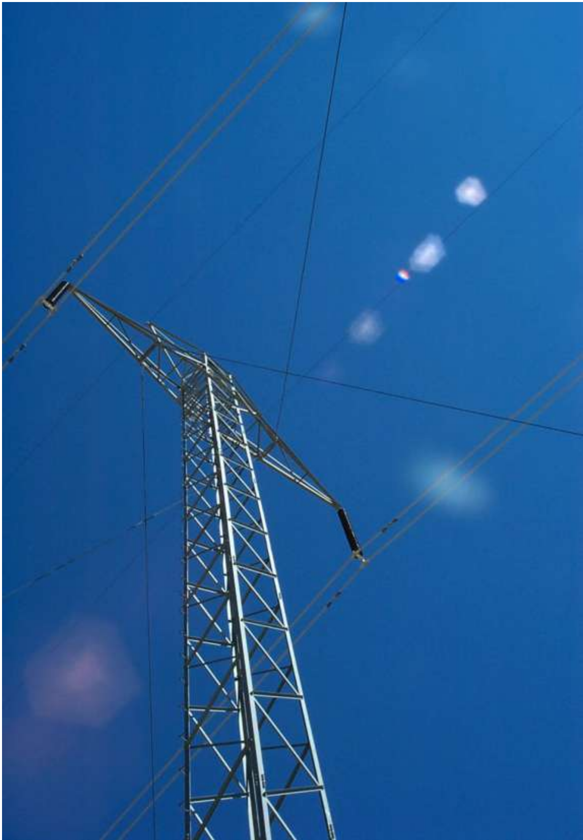
Pacific Intertie 3,100 megawatts, +/-500 kV DC, 1965 LADWP
