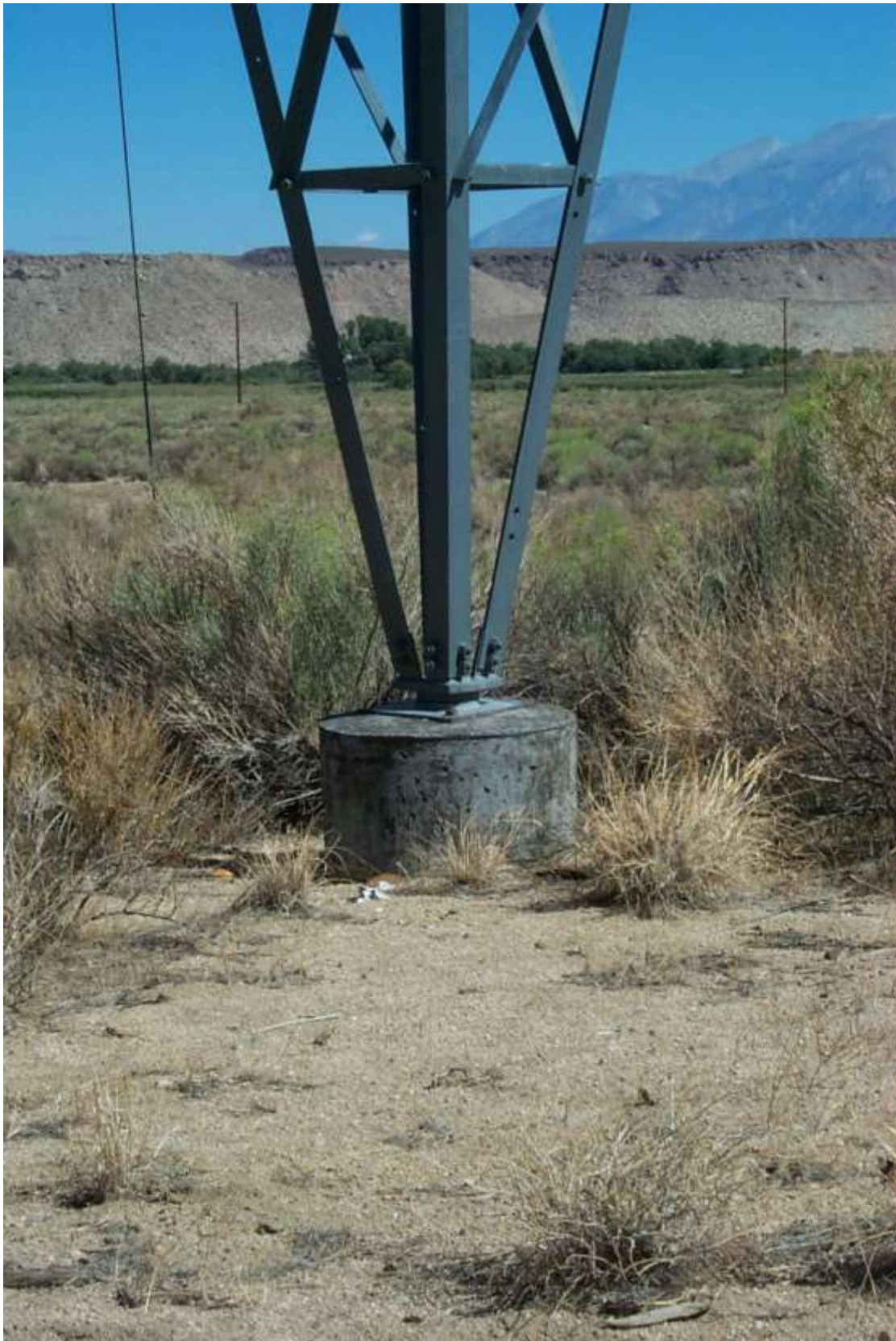
Pylon foundation, Pacific Intertie 3,100 megawatts, 1965 LADWP
