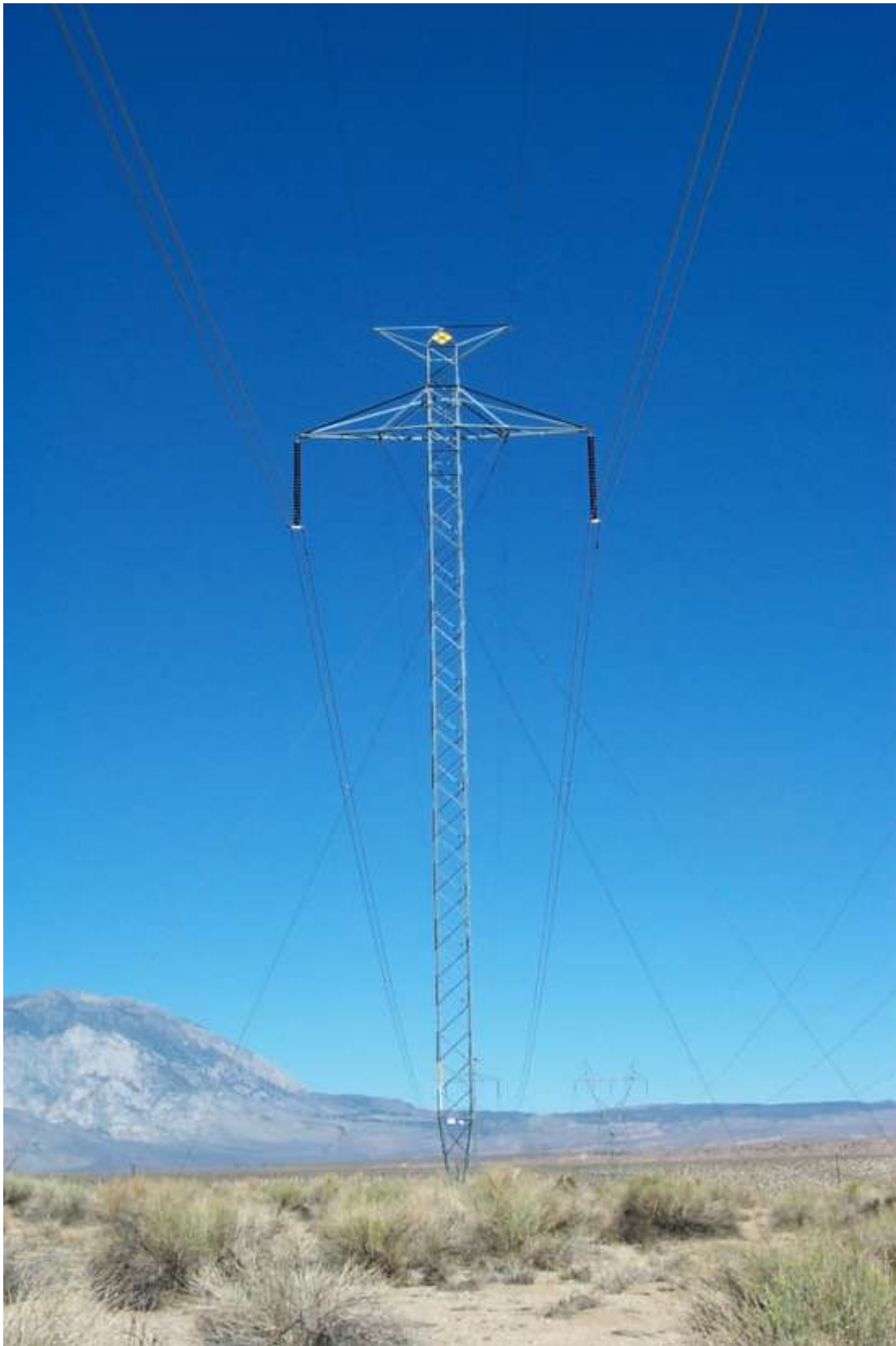
Pacific Intertie 3,100 megawatts, +/-500 kV DC, 1965 LADWP
