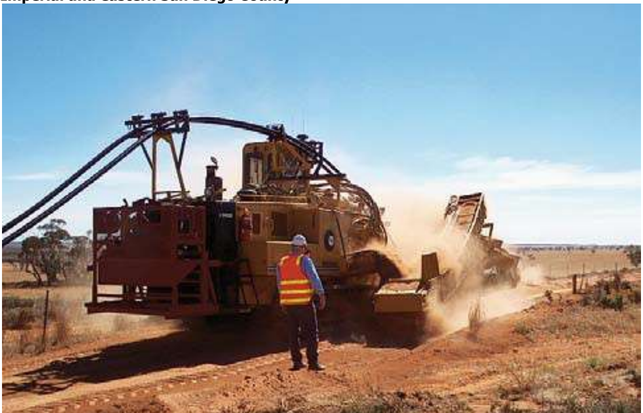
Continuous trenching with underground DC cable installation
