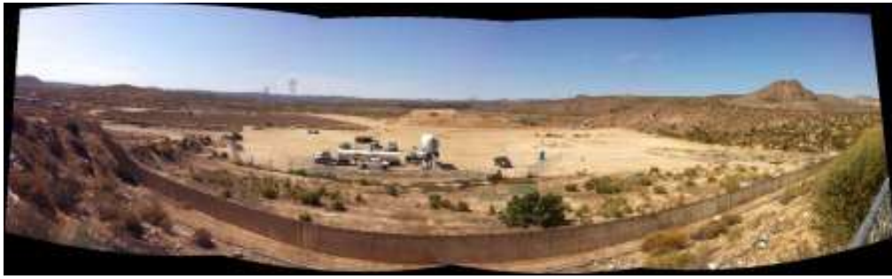
Figure 3: Panoramic view of restoration activities at JVR Yard. ( Link 1 )
