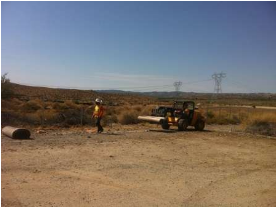
Figure 2: Fence removal at JVR Yard. (Link 1)
