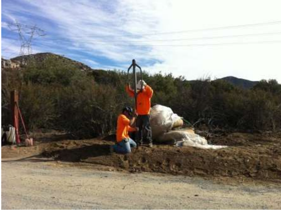
Figure 1: Gate installation at Thing Valley Yard. (Link 2)
