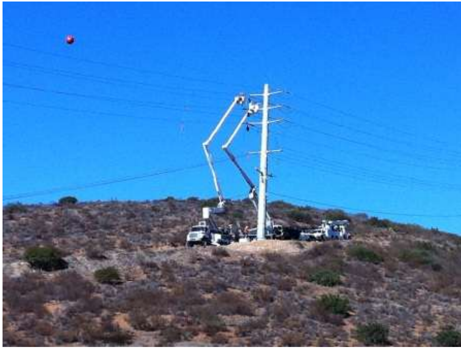
Figure 3: Wire work at Location 11. (Link 5)
