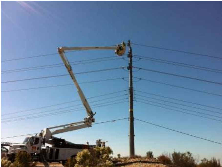
Figure 2: Wire work at Location 9. (Link 5)
