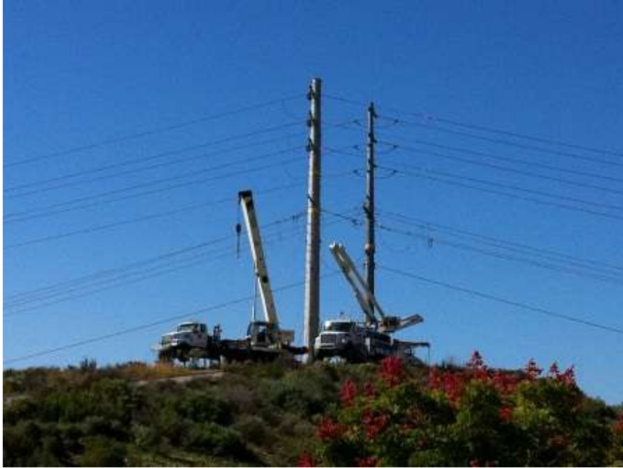
Figure 1: Wire work at Location 8. (Link 5)
