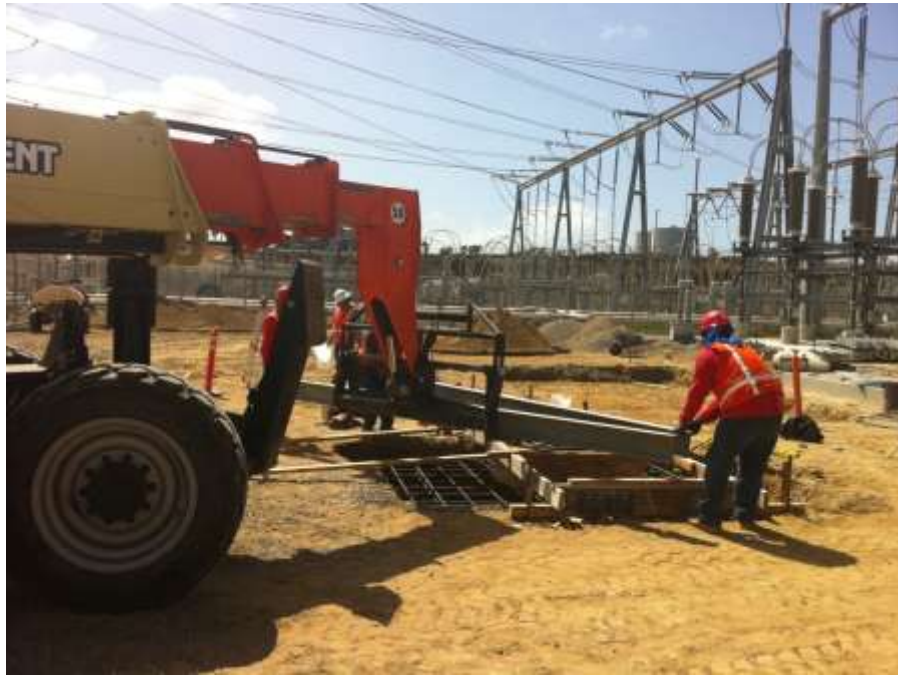
Figure 3: Making forms in preparation for concrete pouring at Encina Substation.
