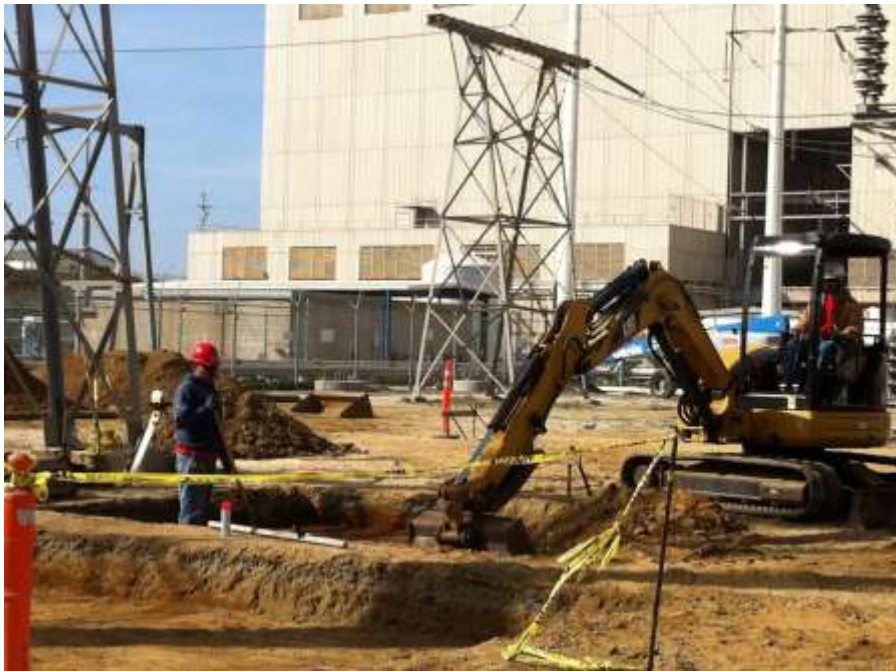
Figure 2: Excavating foundation pads at Encina Substation.
