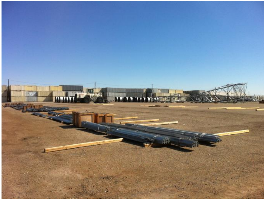
Figure 9: Tower construction at Thomas Yard.
