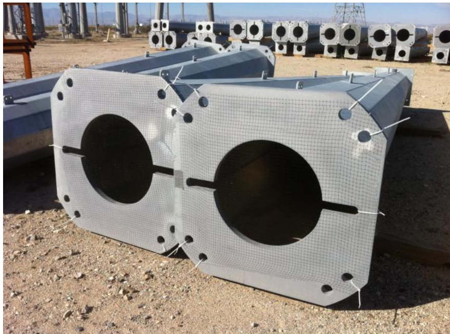
Figure 8: Bird netting installation at Imperial Valley Substation.
