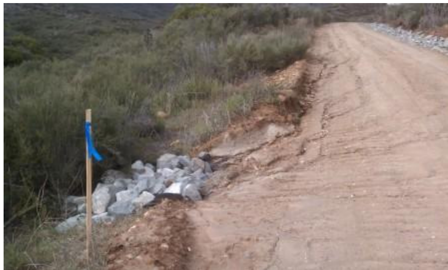
Figure 10: Access road to SWAT Construction Yard.
