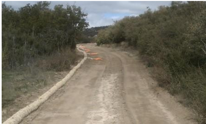
Figure 3: Access road and BMPs to EP 84 & EP 85-2, Link 2.
