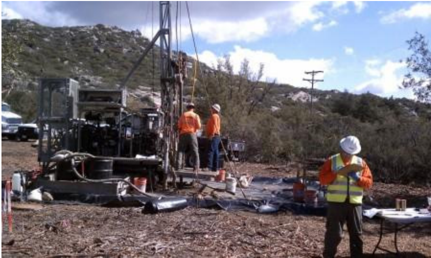
Figure 1: Soil boring at EP 85-2, Link 2.
