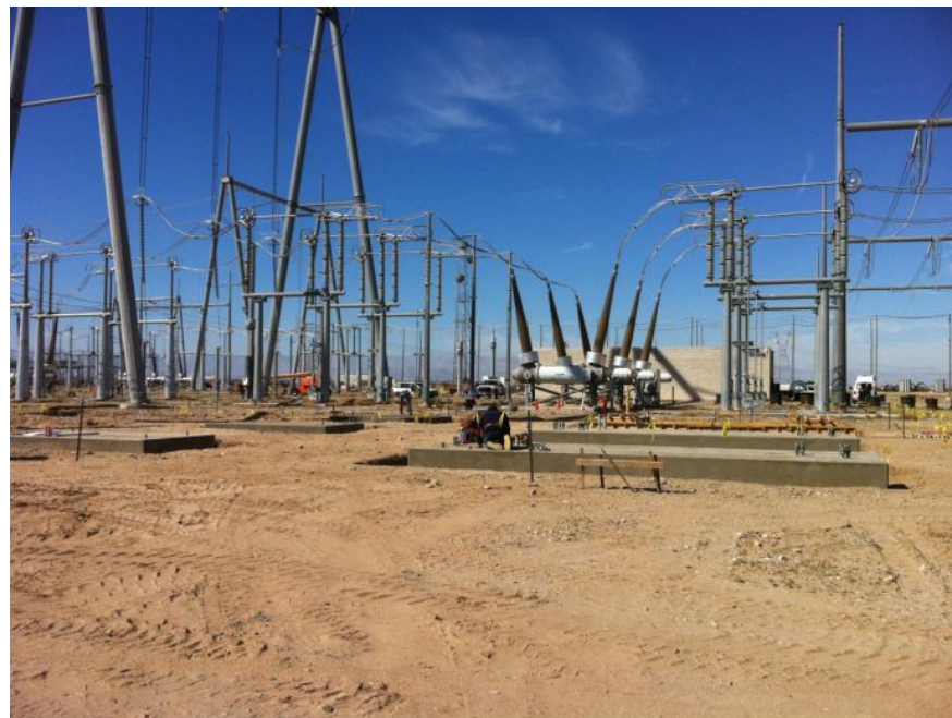
Figure 6: Foundation work at Imperial Valley Substation.
