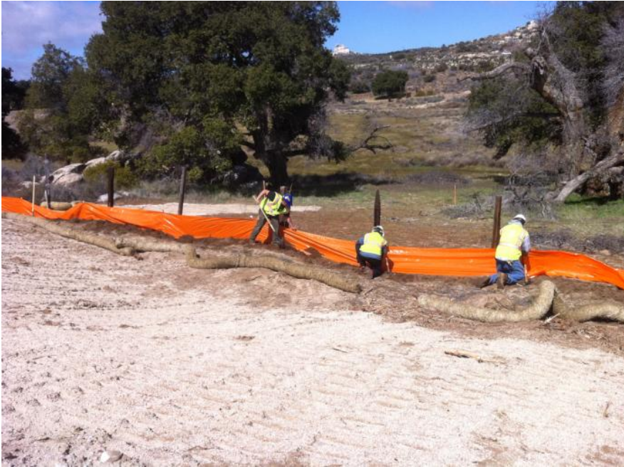
Figure 2: BMP repair at EP 220 within Red Tailed Hawk nest buffer, Link 1.
