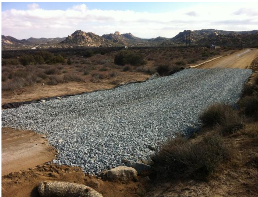
Figure 4: Implementation of BMPs; rocked dip section along access road, Link 2.
