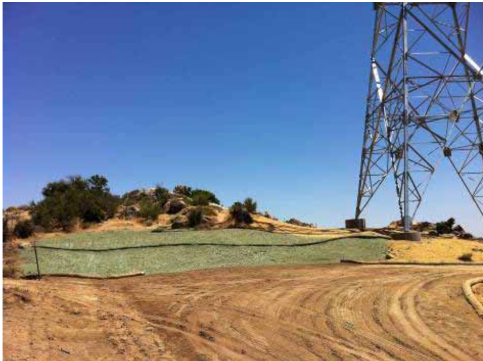
Figure 5: Hydromulch application at EP219-1, Link 1.
