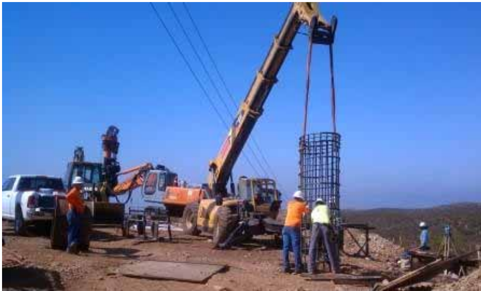
Figure 4: Installation of rebar at CP19-1, Link 5.
