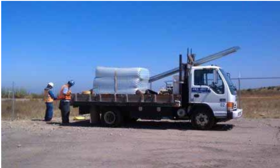
Figure 8: Fence installation at Sycamore Yard, Link 5.
