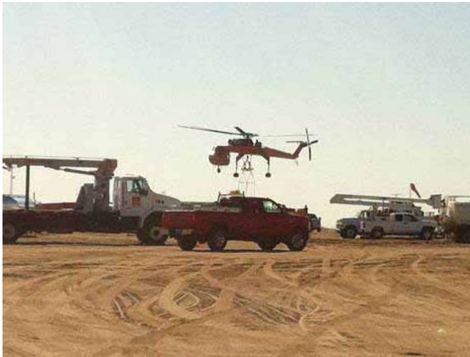
Figure 2: Erickson Sky Crane test flights at Plaster City Yard, Link 1.
