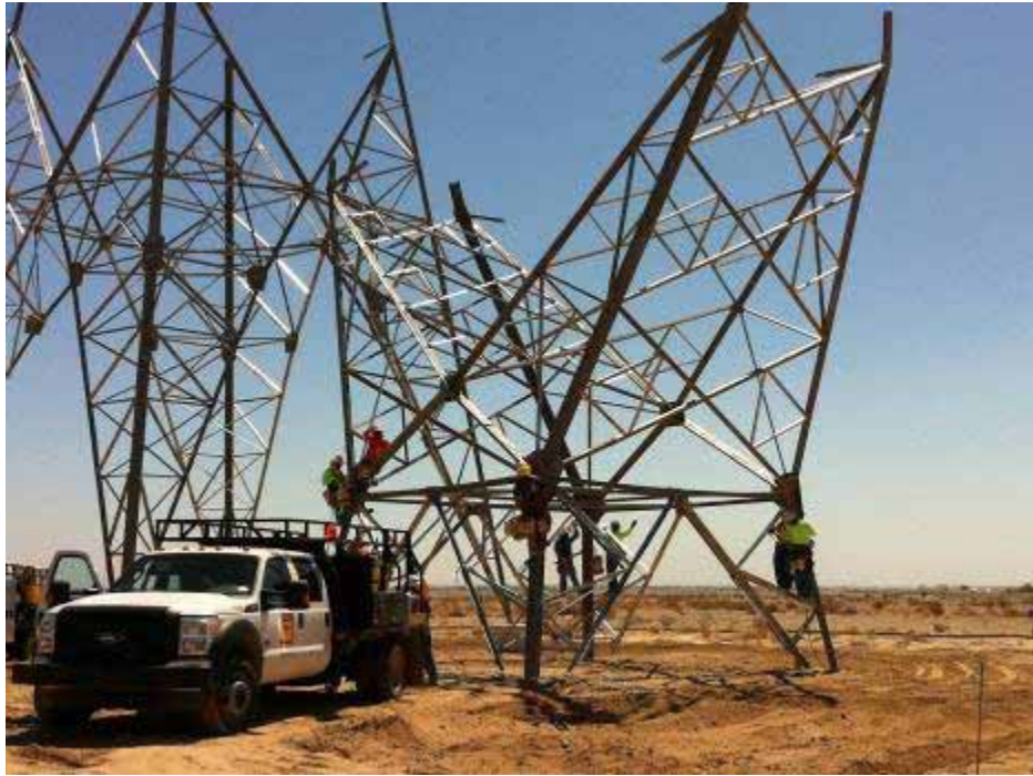
Figure 1: Conventional tower assembly at EP341, Link 1.
