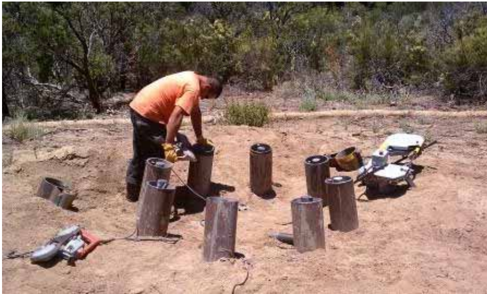
Figure 3: Trimming micropiles at EP 85-2, Link 2.
