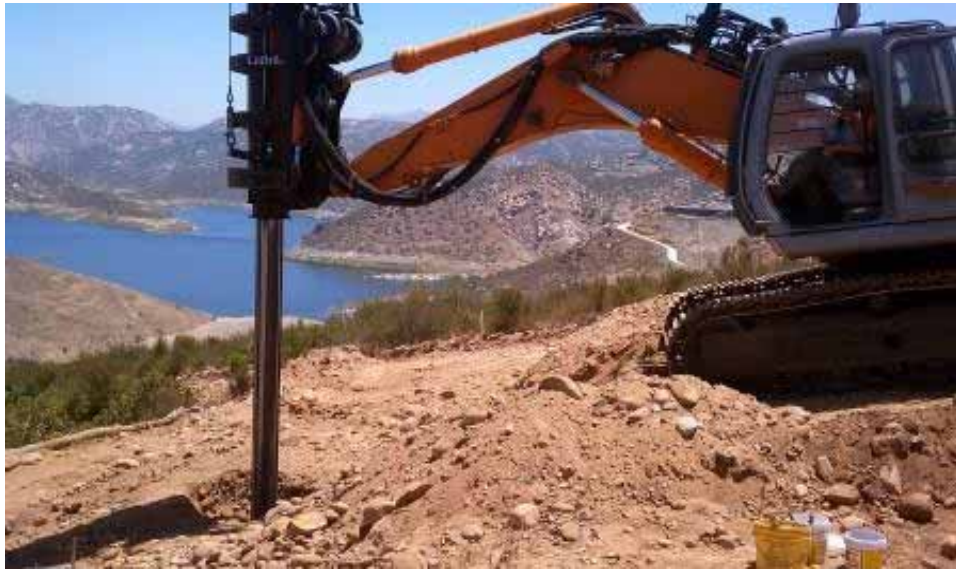
Figure 3: Conventional drilling at CP 41-2; San Vicente Reservoir in the background. (Link 5)
