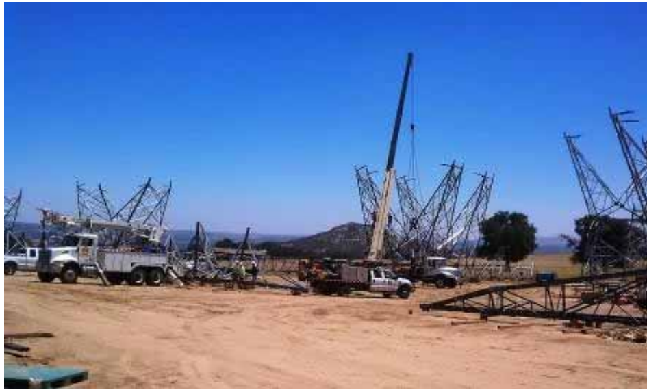
Figure 7: Tower assembly at Bartlett-Hauser Construction Yard. (Link 5)
