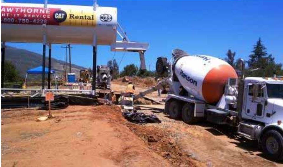
Figure 2: Installation of Vault 20R. (Link 4)
