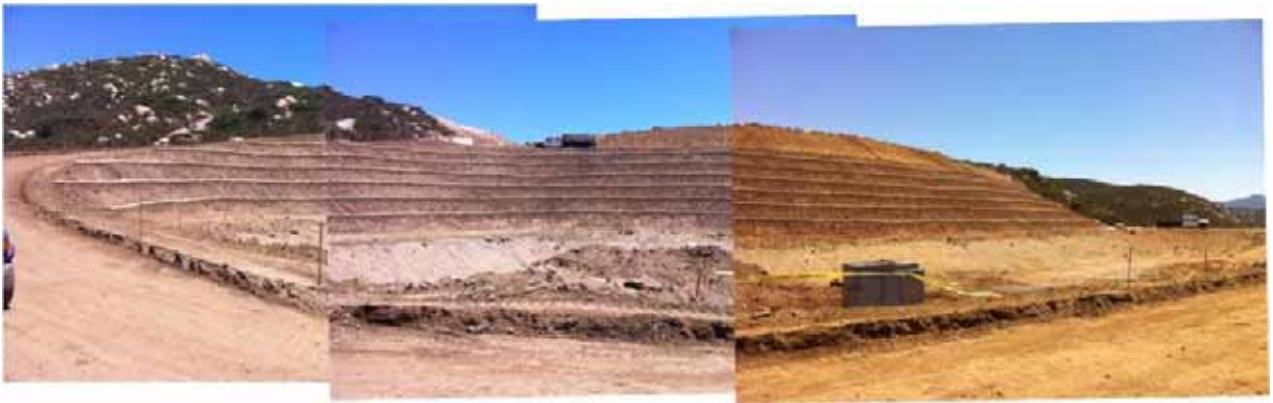
Figure 5: BMP installation on finished slope at Suncrest Substation, Link 3.
