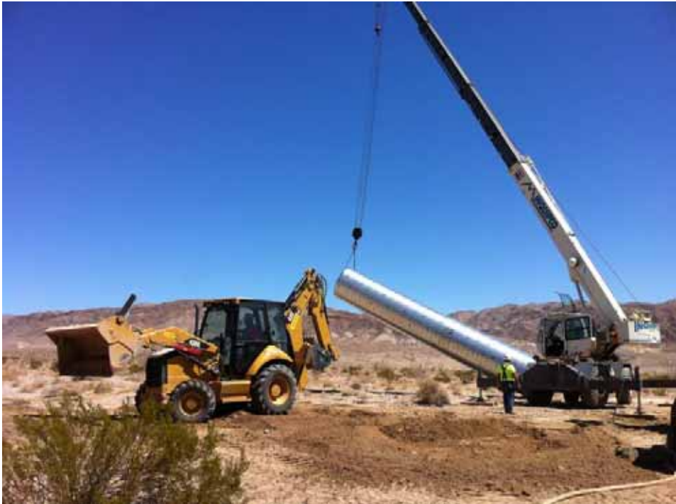
Figure 1: Setting corrugated pipe to stabilize the hole at EP298, Link 1.
