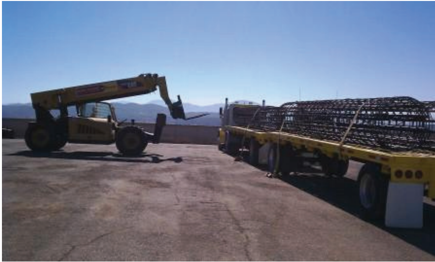
Figure 12: Delivery of rebar at Sycamore Construction Yard. (Link 5)
