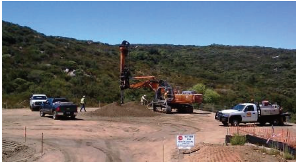
Figure 3: Drilling at CP95-1. (Link 5)
