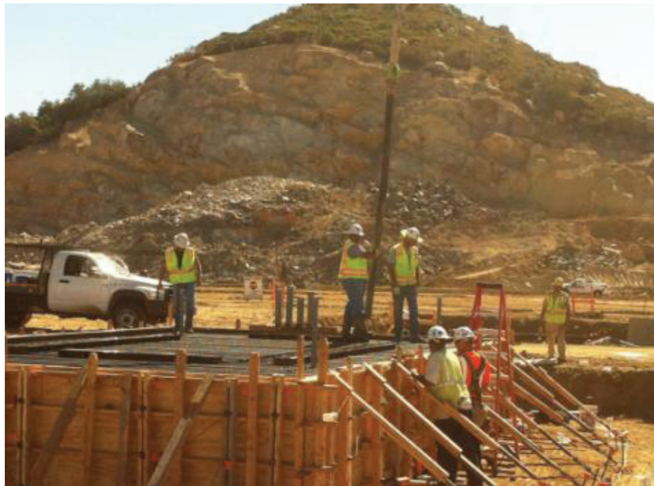
Figure 8: Foundation pouring at Suncrest Substation. (Link 3)
