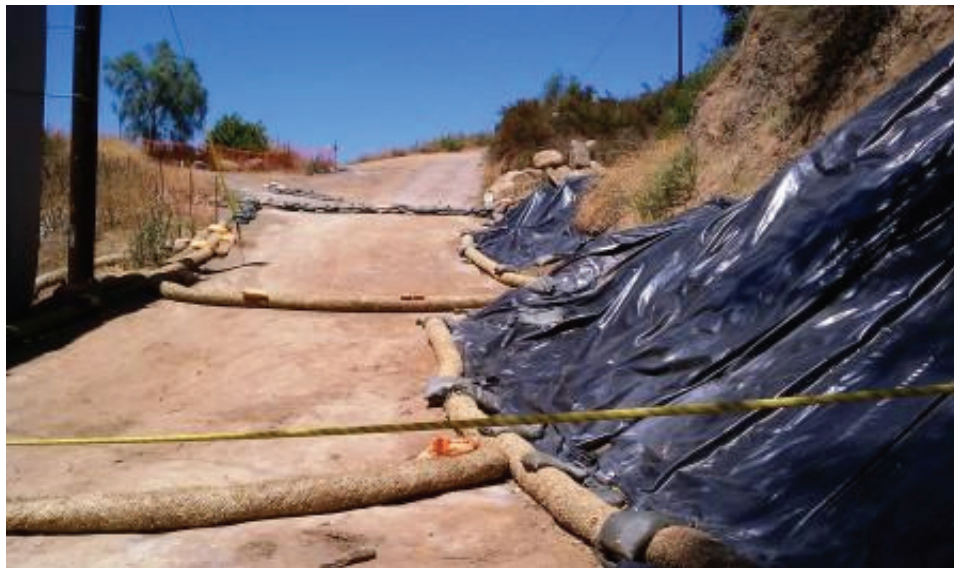
Figure 6: BMPs at Bauer Bridge. (Link 4)
