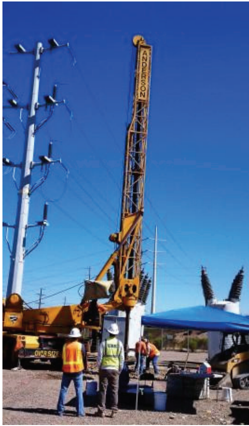
Figure 9: Drilling for a tower foundation at Sycamore Substation. (Link 5)
