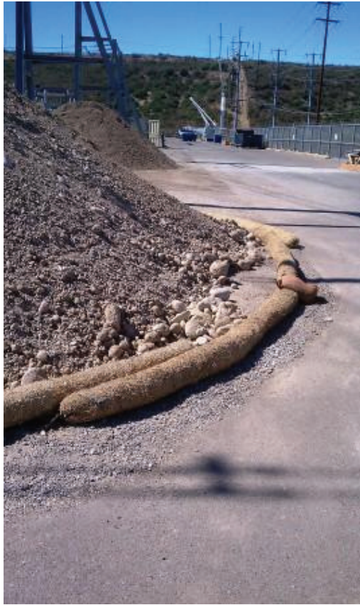
Figure 10: BMPs for spoil piles at Sycamore Substation. (Link 5)
