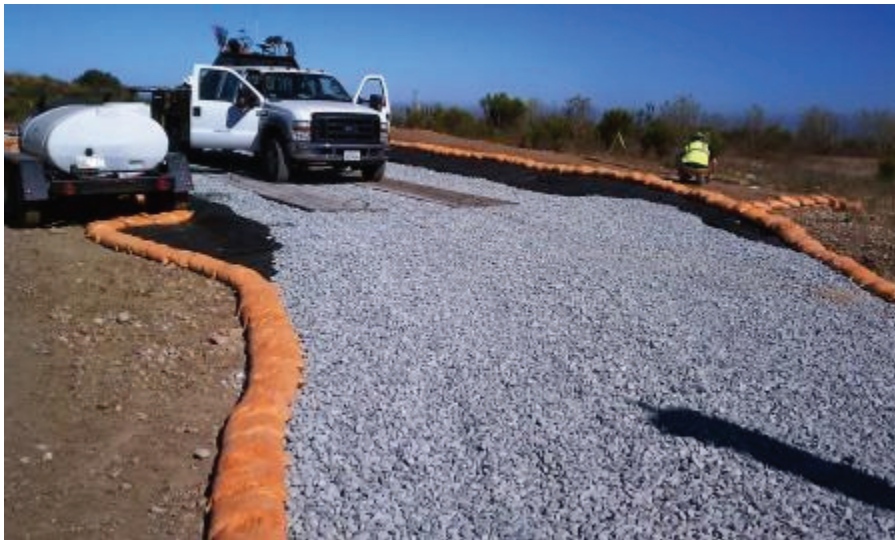
Figure 13: Wash station installation at Sycamore Construction Yard. (Link 5)
