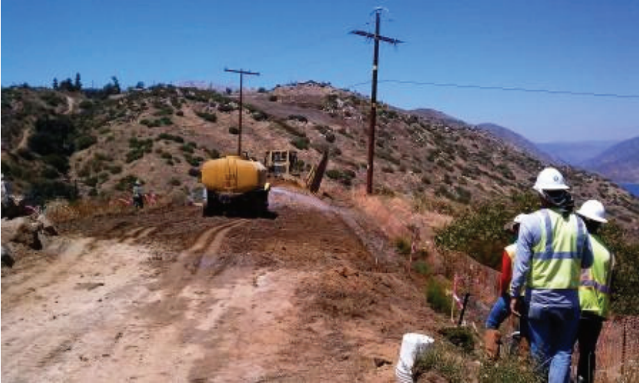
Figure 1: Grading occurring at the Slay property. (Link 4)
